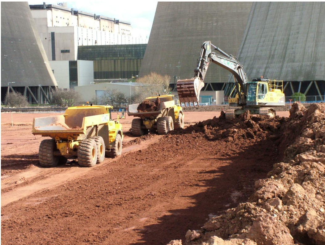
Plate 11: Work in progress on new station site, looking east
