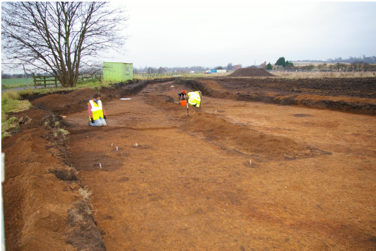
Plate 3: Work in progress on Access Road trench, looking north-west
