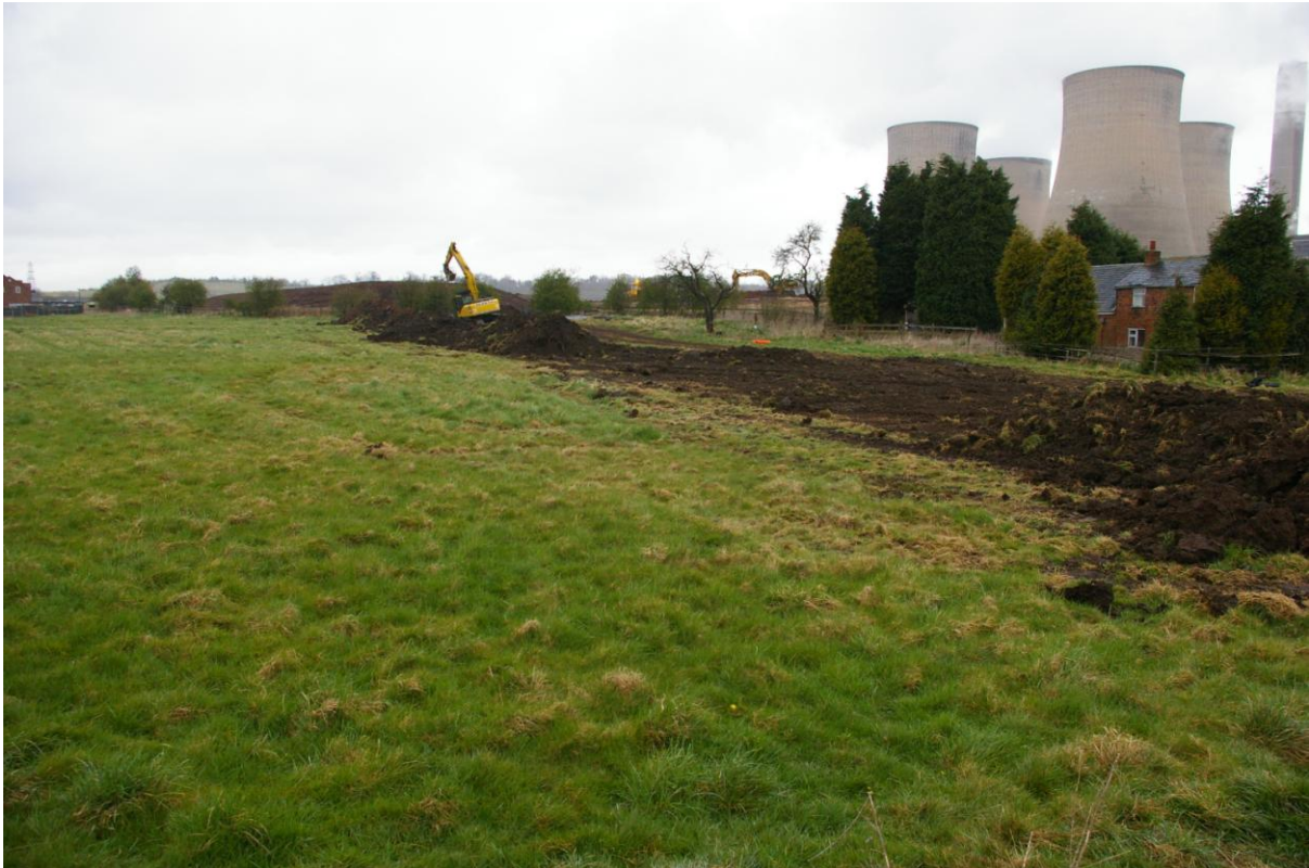
Plate 13: Topsoil stripping in Field 3, prior to trenching for drainage, looking north-east
