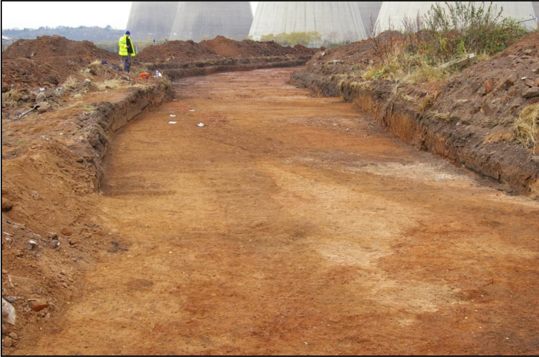
Plate 2: Haul Road trench, after stripping, looking north-east
