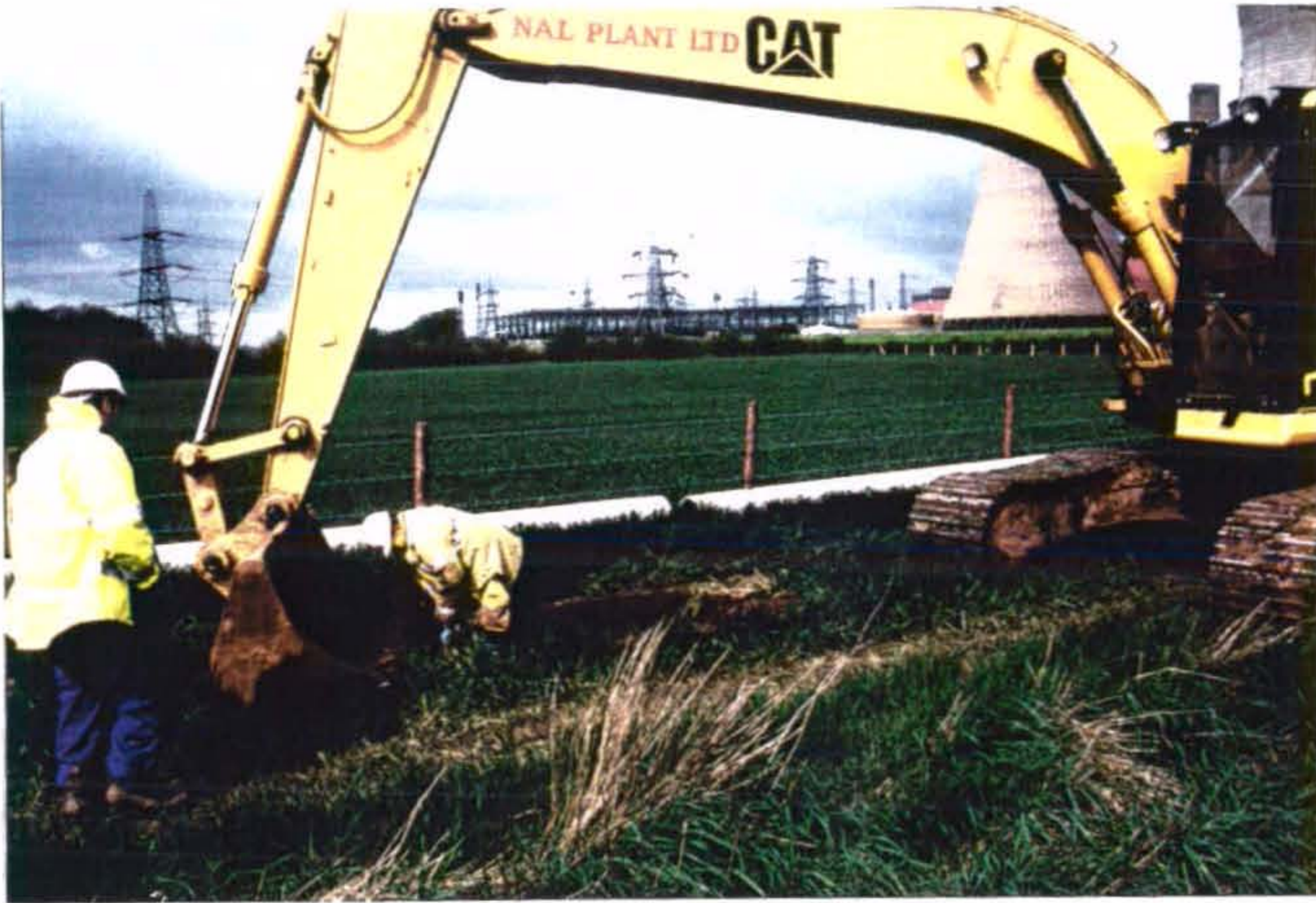
Plate 1 Excavation in progress, Pipeline A
