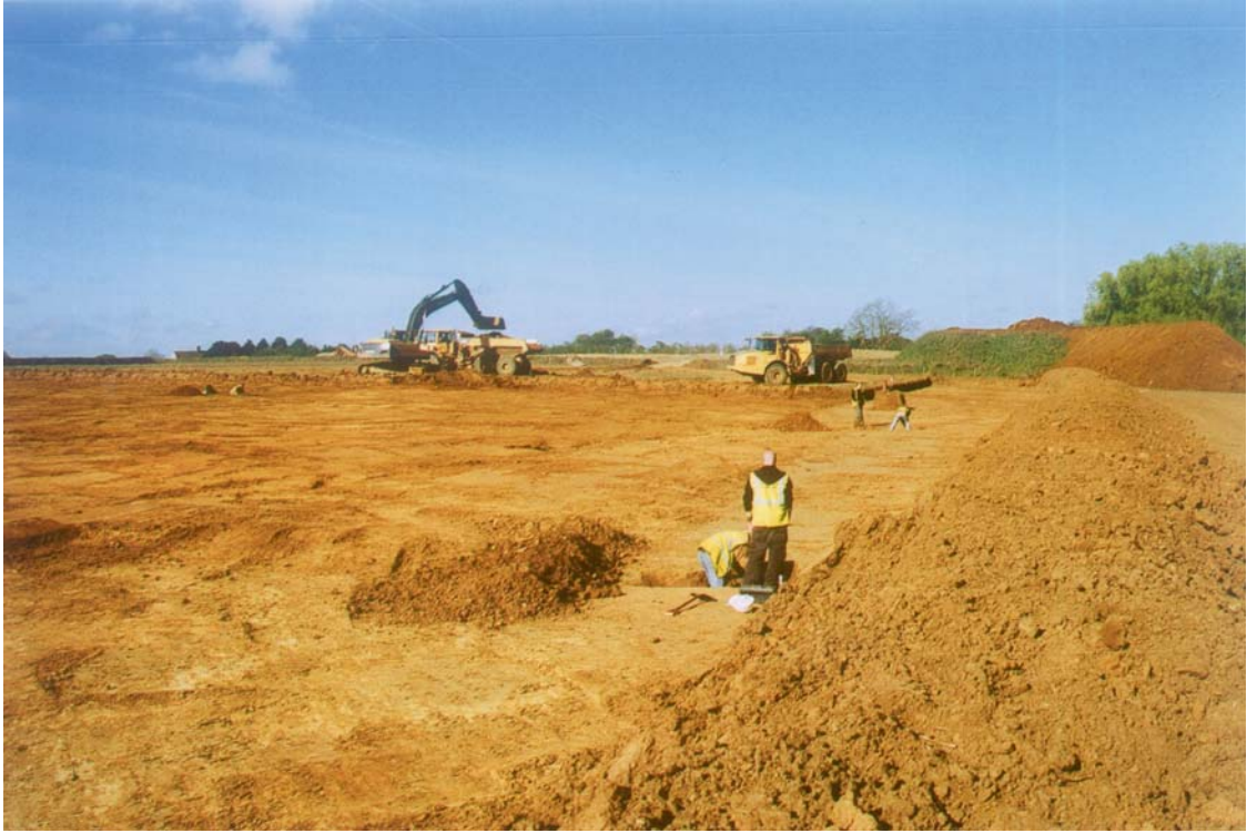
Plate 1. Working shot over stripped area, looking west
