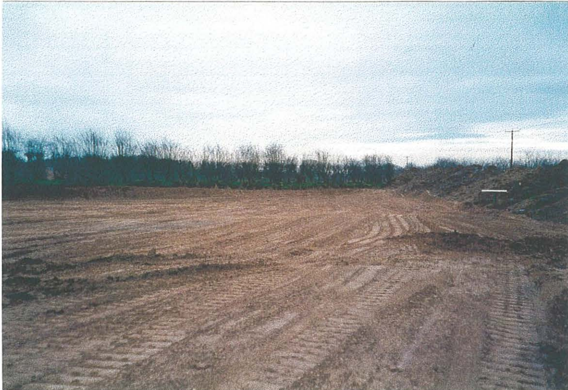
Plate 1. South-western corner of site after topsoil stripping. Facing South-west.
