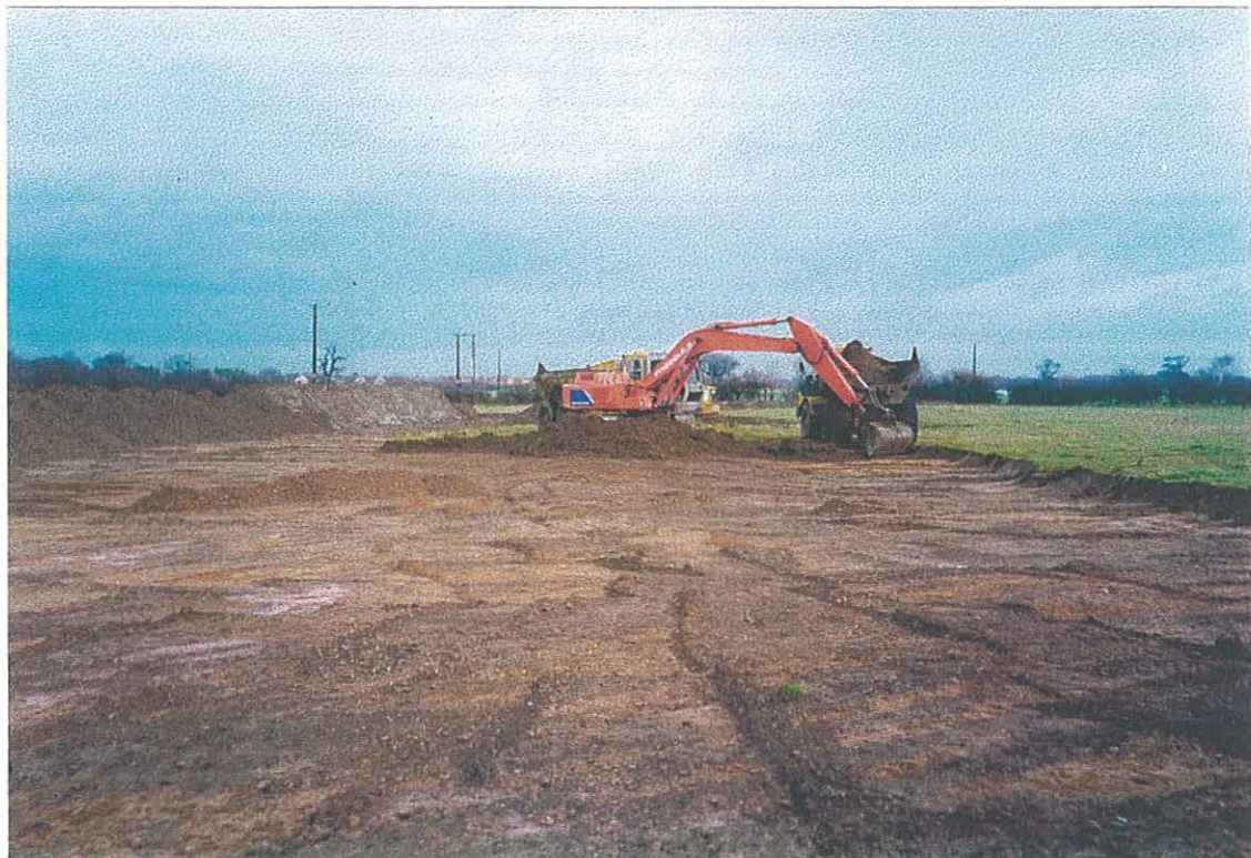
Plate 2. Western area of site during topsoil stripping. Facing North.
