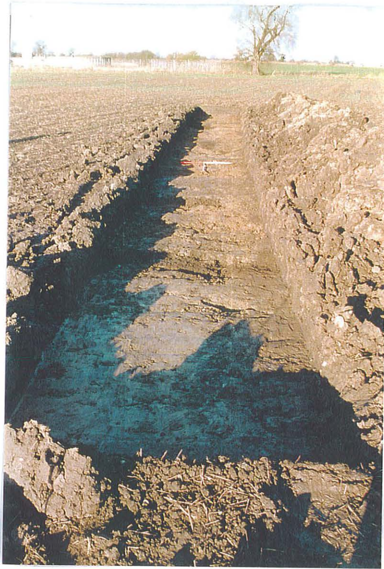
Plate 23. Overall View of Trench 12. Facing North.
