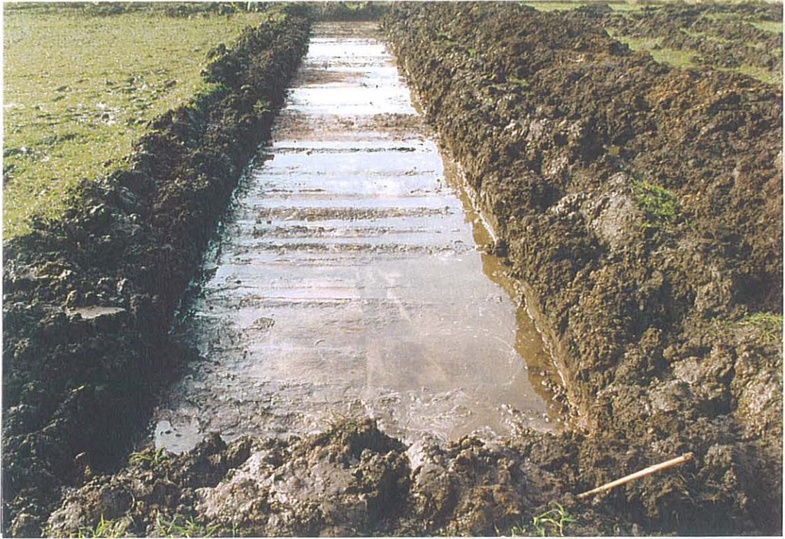
Plate 13. Overall View of Trench 4A. Facing South-west.
