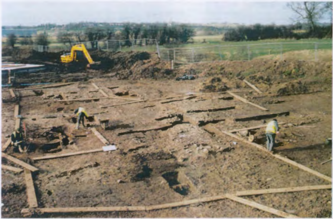
Plates 1 and 2 Overall site shots showing extent of main excavated area
