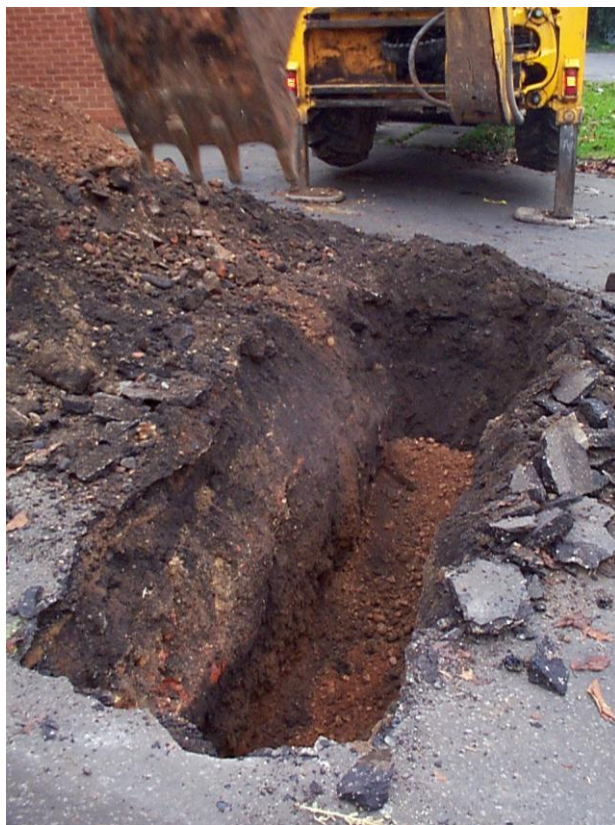
Fig. 6: Excavation of test pit 3
