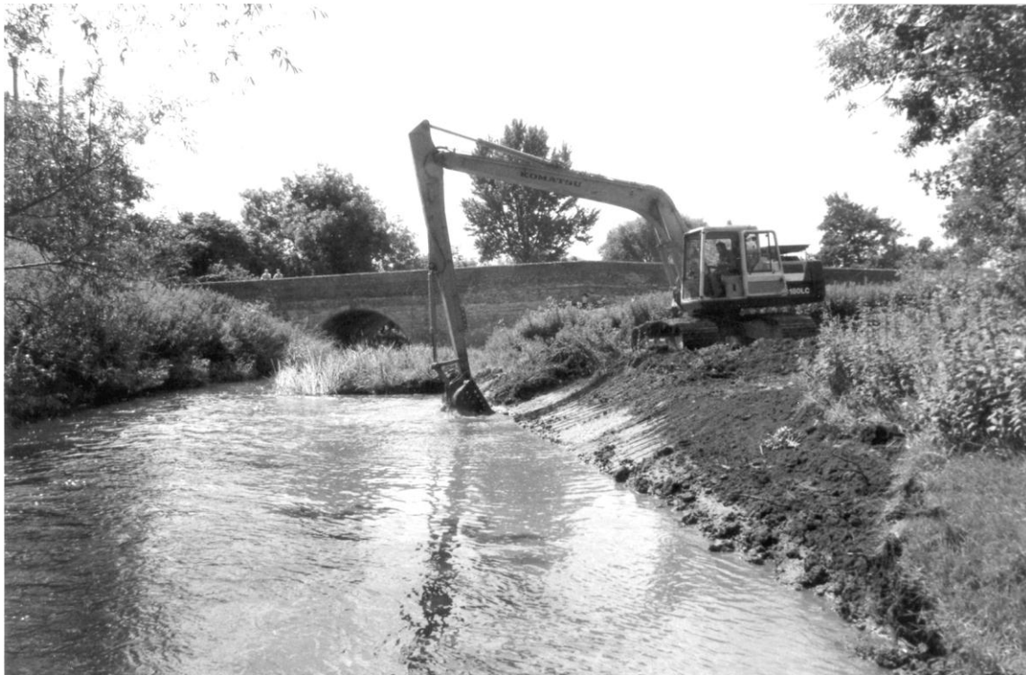
Fig. 6: Removal of silt deposits at Oversley Bridge (Area 1)
