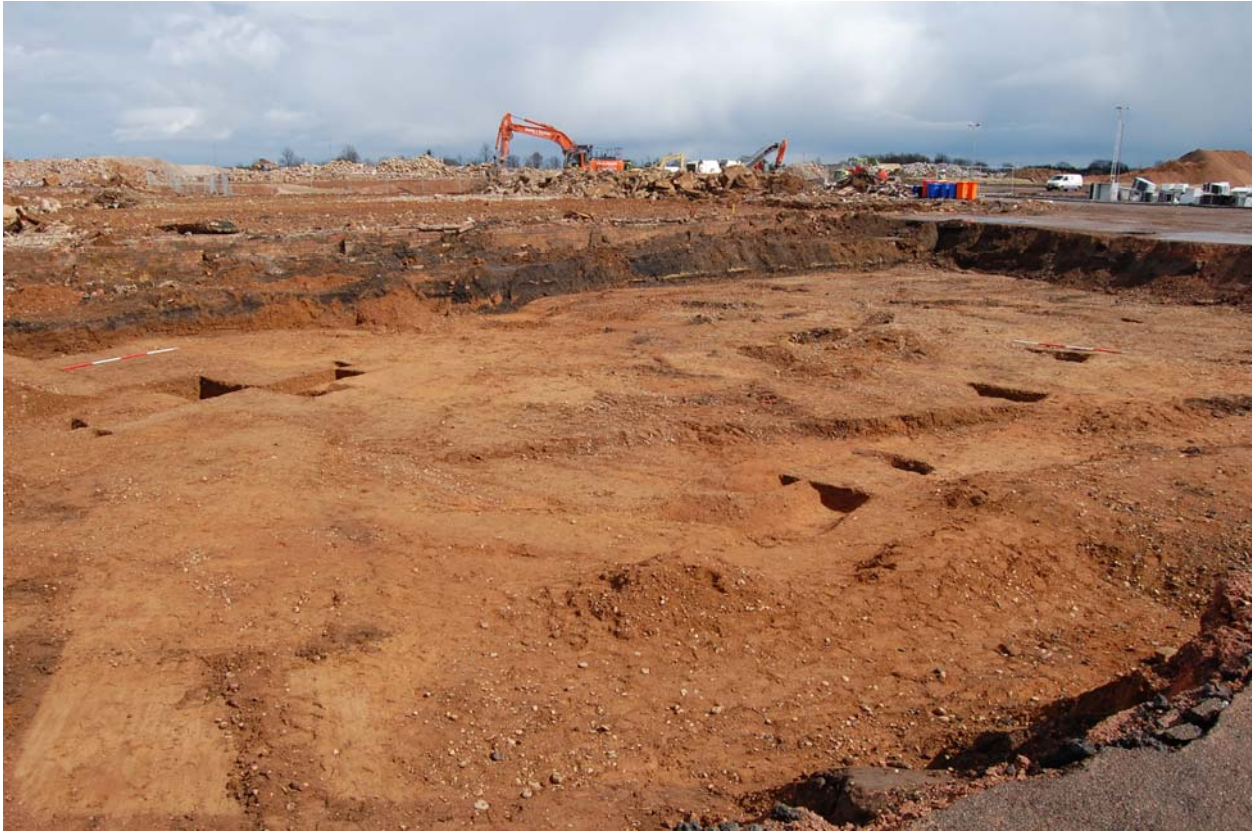
Fig. 4: The site looking east
