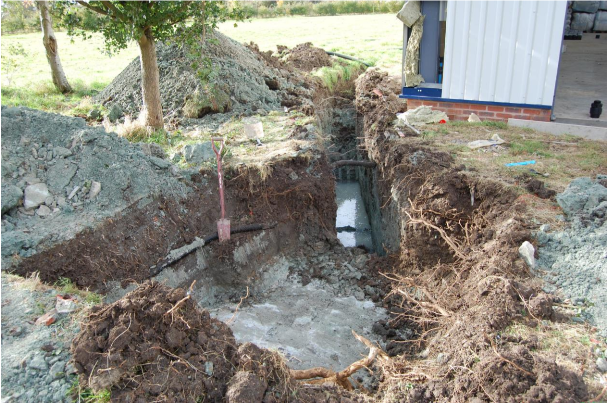
Fig. 6: Tank trench and drainage trench
