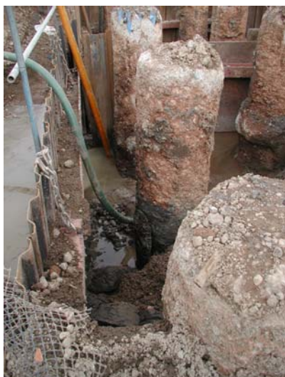
Plate 16: Wooden pile with poured concrete pile immediately adjacent
