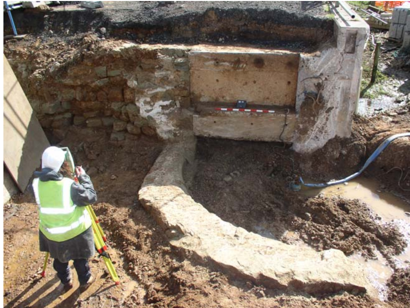
Plate 15: Bridge spandrel and wing wall (Section BO)
