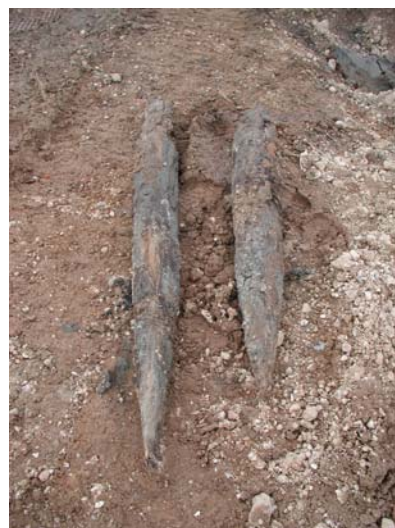
Plate 17: Two wooden piles removed by contractors
