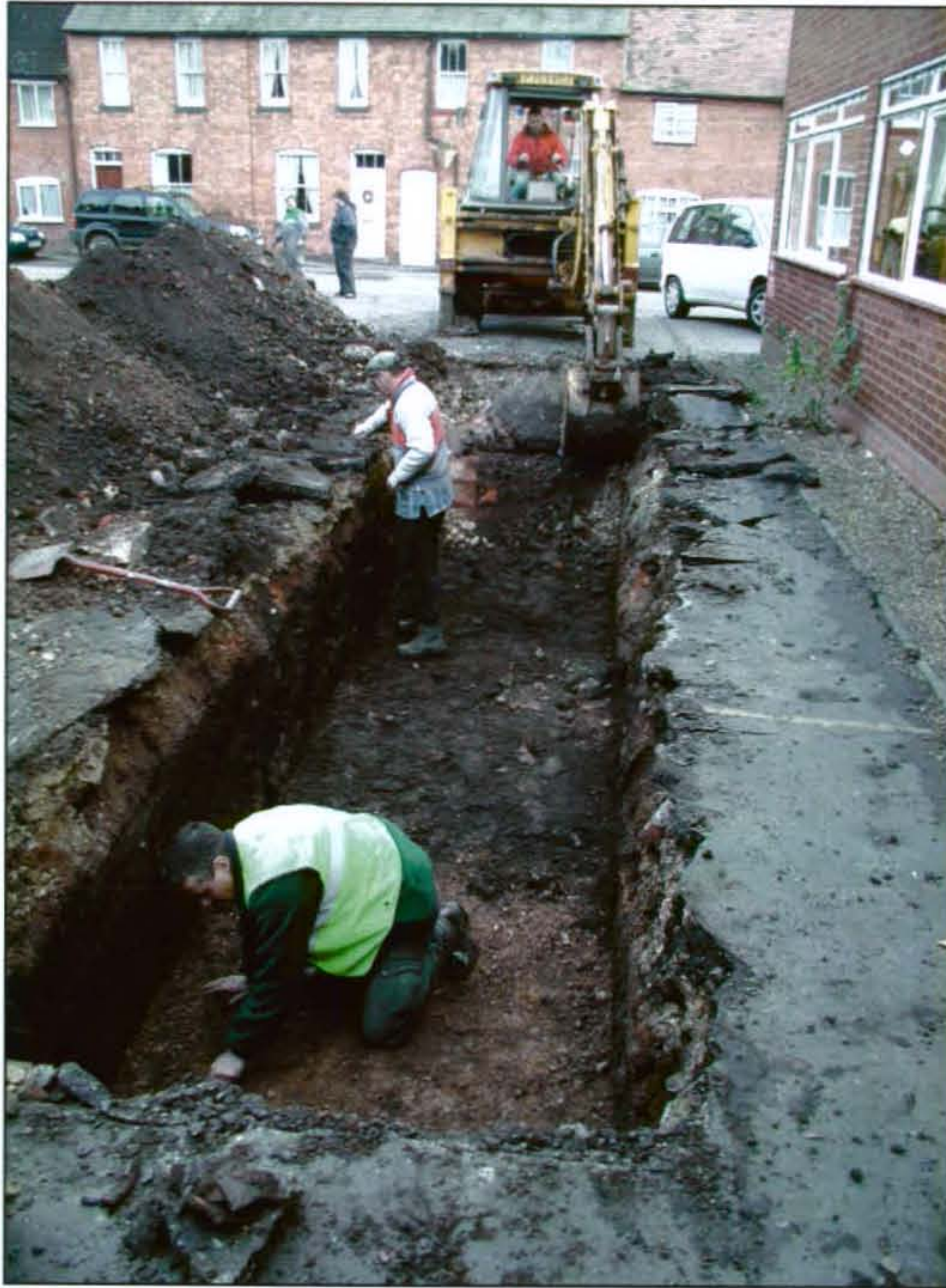
Fig. 12: Trench 8 during excavation of gravel surface (816)
