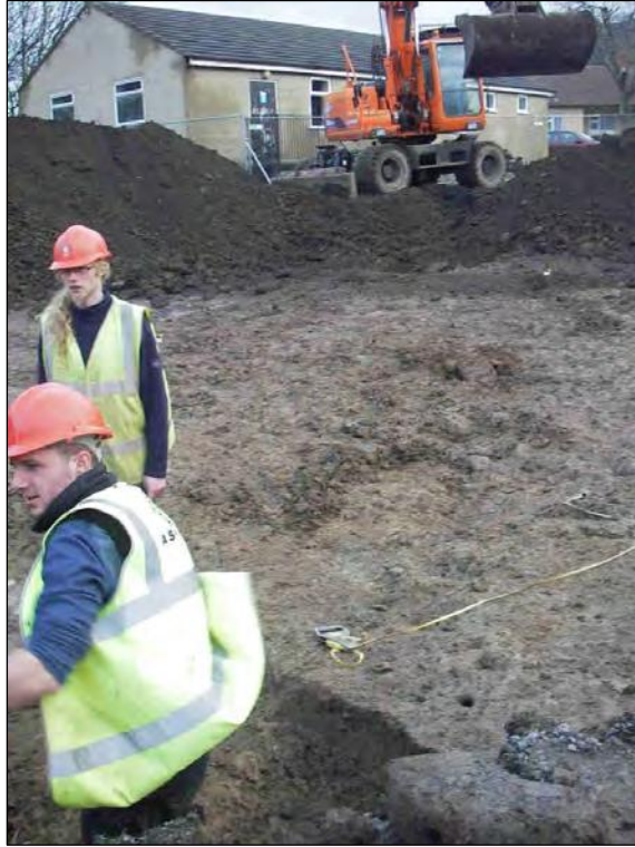
Plate 9: Working shot during the excavation of Area A, looking northeast
