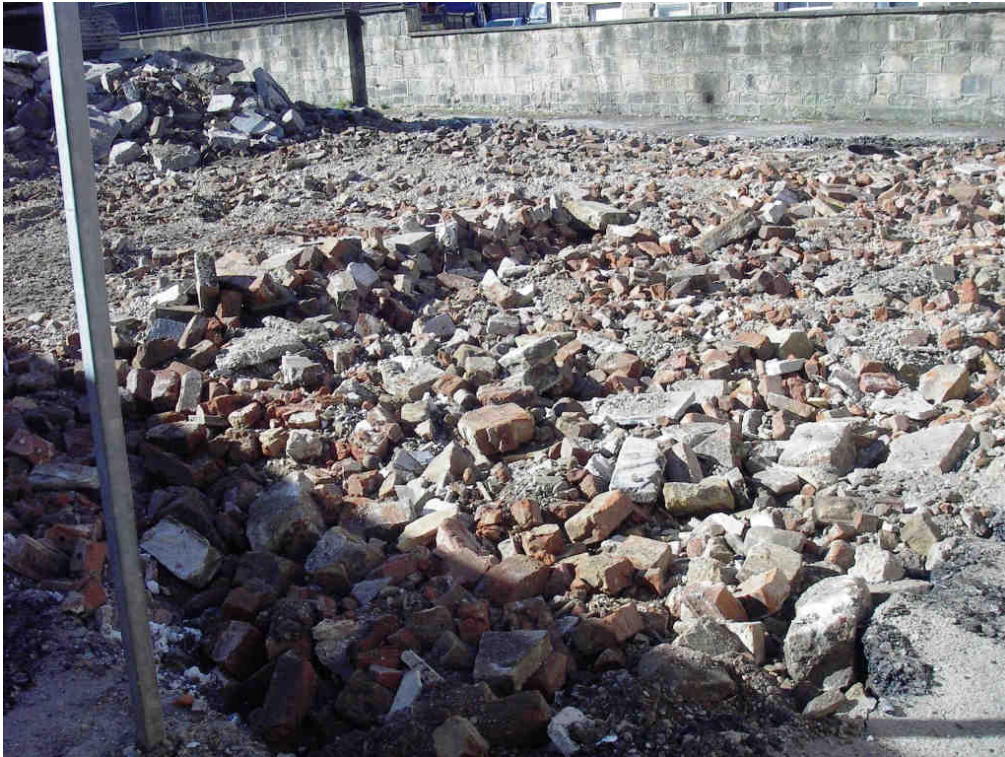
Plate 10: Watching brief during the demolition of the court building, Area B,
