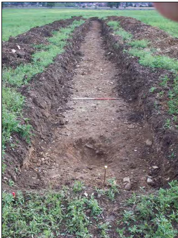
Plate 16. Trench 15, looking north-east
