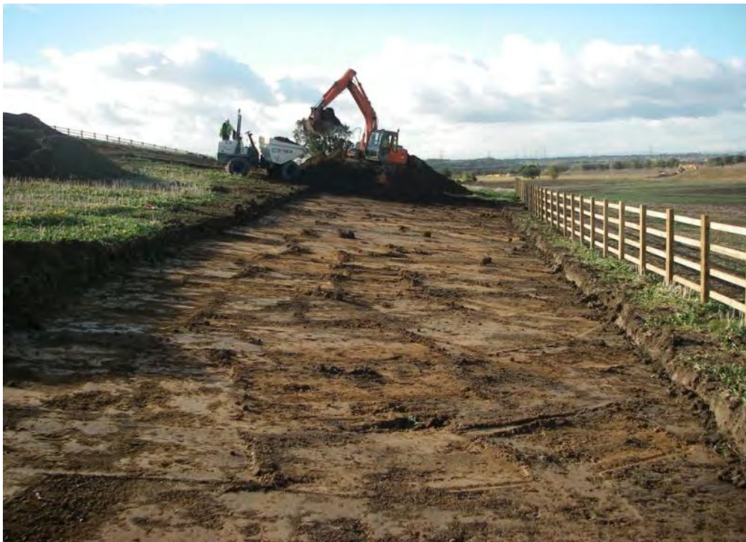
Plate 6: Stripping the excavation area around Trench 7, looking southwest
