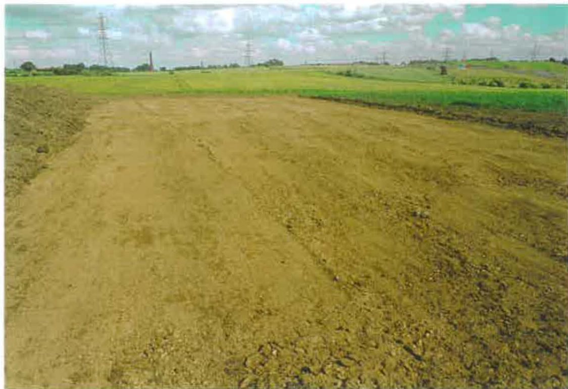
Plate 1. Areas A and B Environs. Prior to excavation. Facing East.
