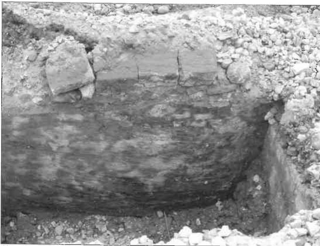
Plate 18. Ground reduction area, tank (530), looking west.
