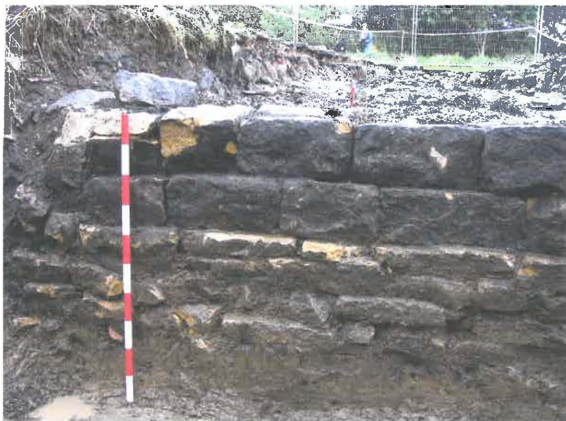
Plate 5 , Facing east, part of wall 3015, showing the upper two courses of gritstone blocks above a small off-set course and three foundation courses
