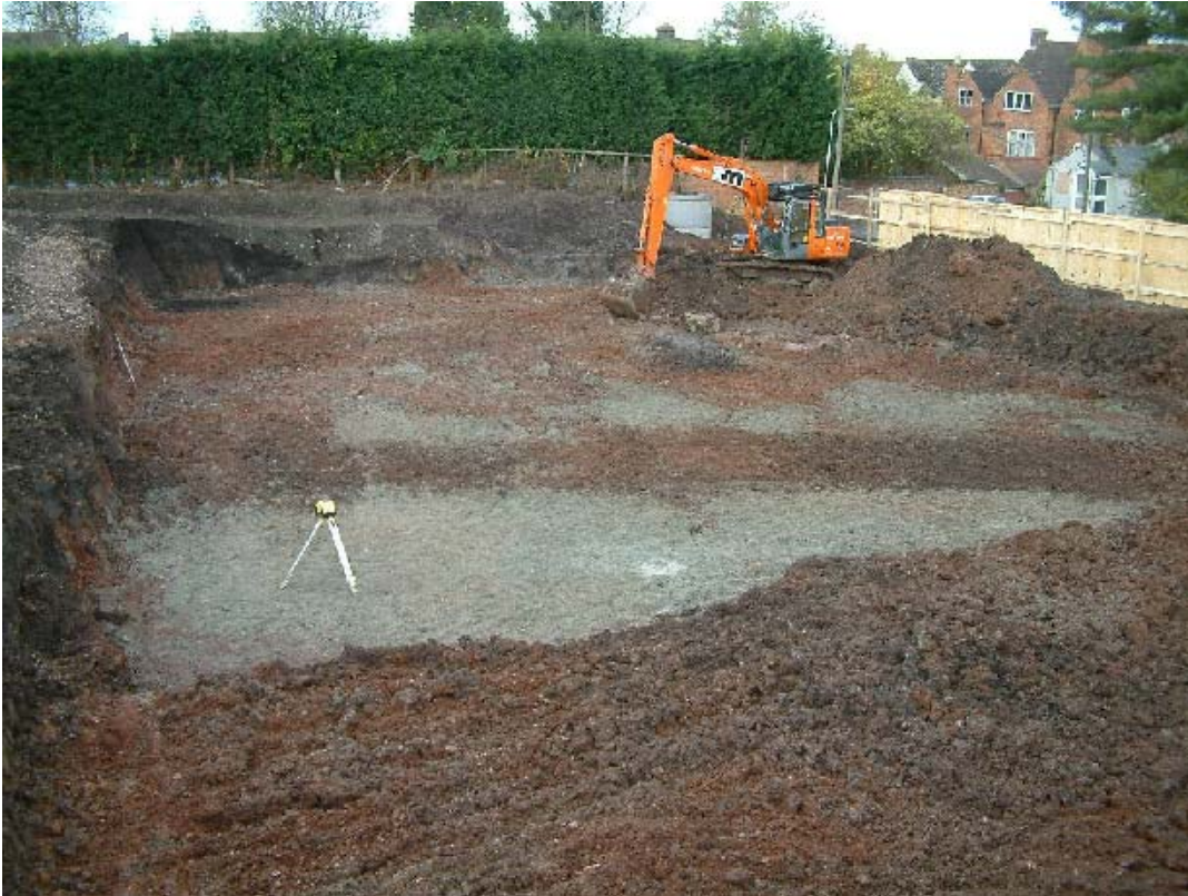
Plate 14: Site after contractor machining. Note base of the large ditch still visible across the site
