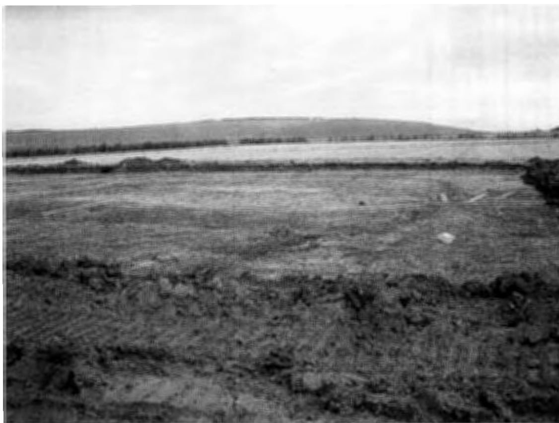
Plate 2: Area 3, as stripped, view north
