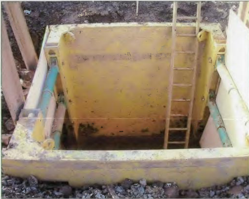
Plate 5. Trench 4 box shoring.
