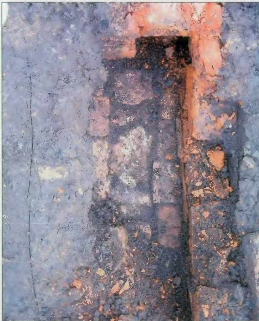
Plate 6. Trench 4, showing culvert [4004].
