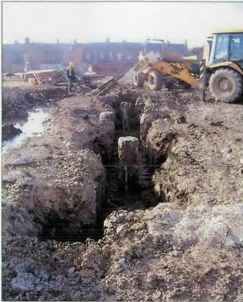
Plate 1. General working shot of Trench 1.
