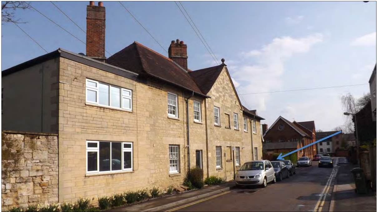
Fig 3: 'The manor', site of the 1824-35 Summertown Workhouse, looking south along Mayfield Road's eastern frontage. Note the laundry application site (arrowed) just beyond.
