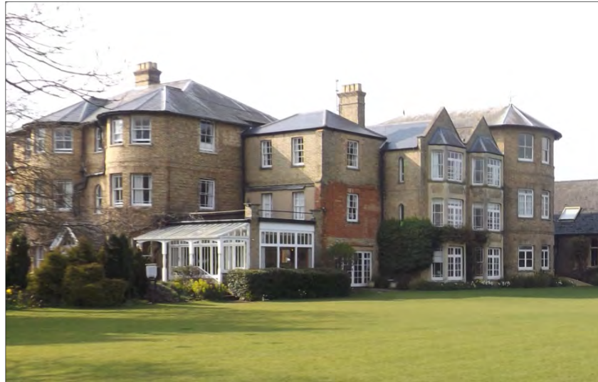
Fig 9: The main school core, viewed from the south-east
