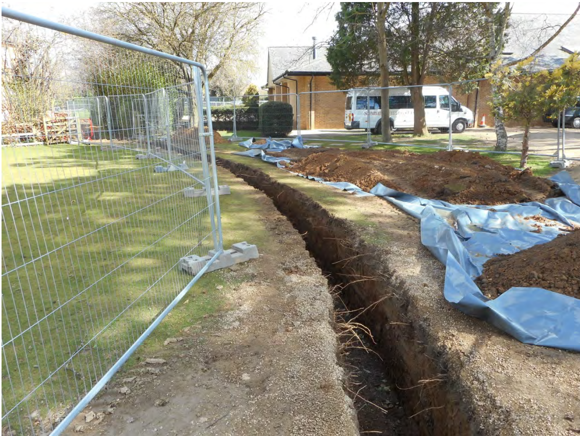
1. Service Trench, looking north-east
