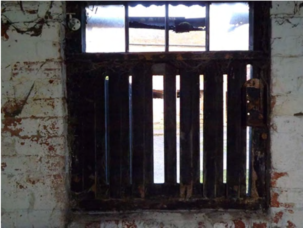
IBC 27: The stables; a sliding ventilation shutter of offset slats
