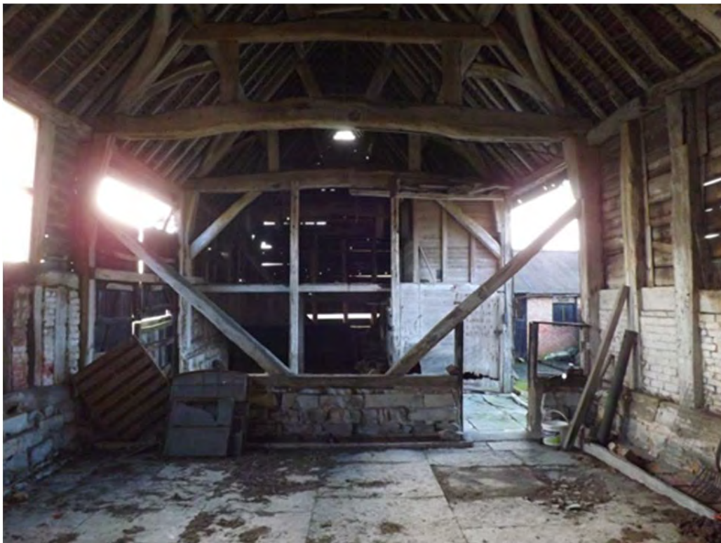
IBC 16: Barn interior, looking south
