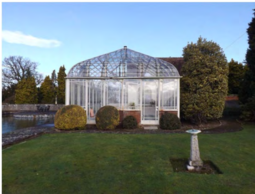
IBC 40: The hipped south gable with two doors
