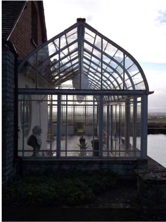
IBC 39: Pool house annexe, north gable; here its greenhouse basis is most easily seen
