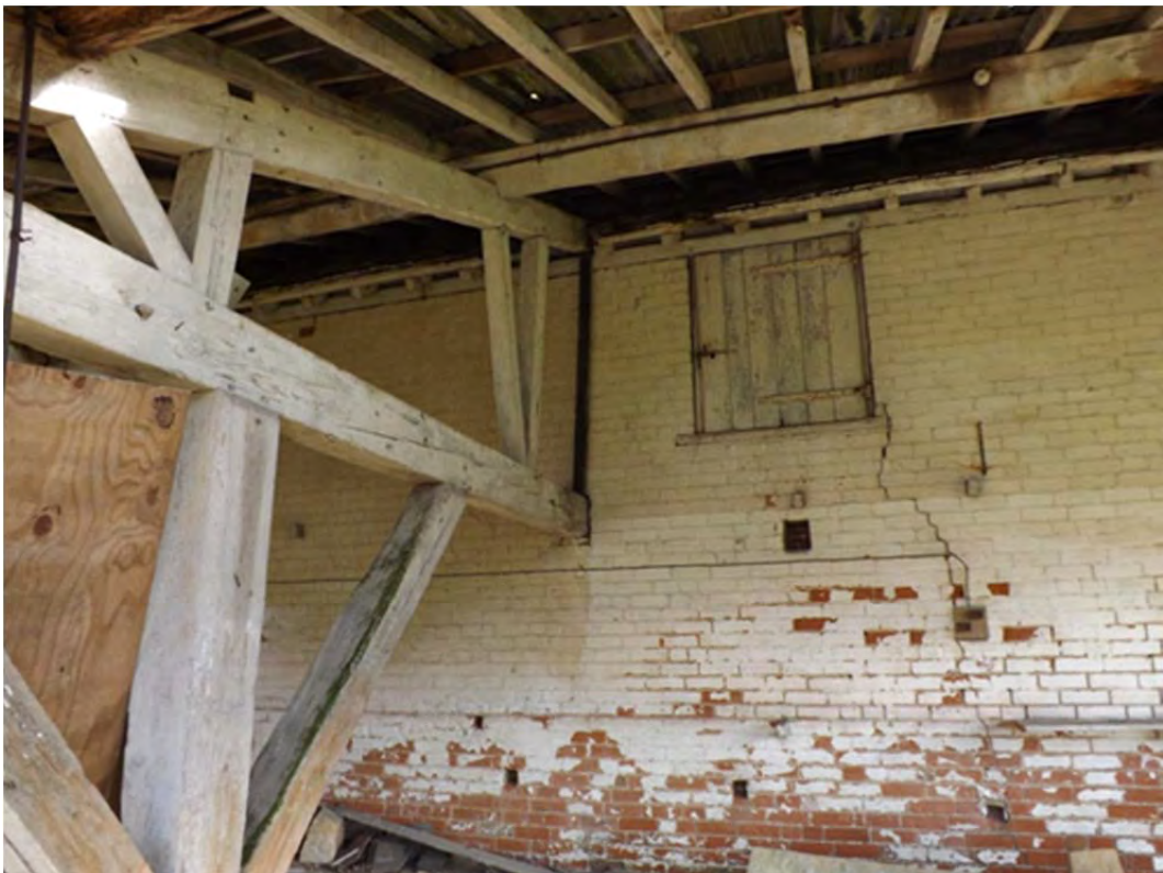
IBC 30: 20th-century lean-to addition to the stable rear (west)
