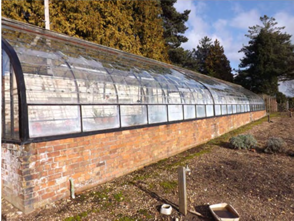
IBC 35: View along the greenhouse exterior
