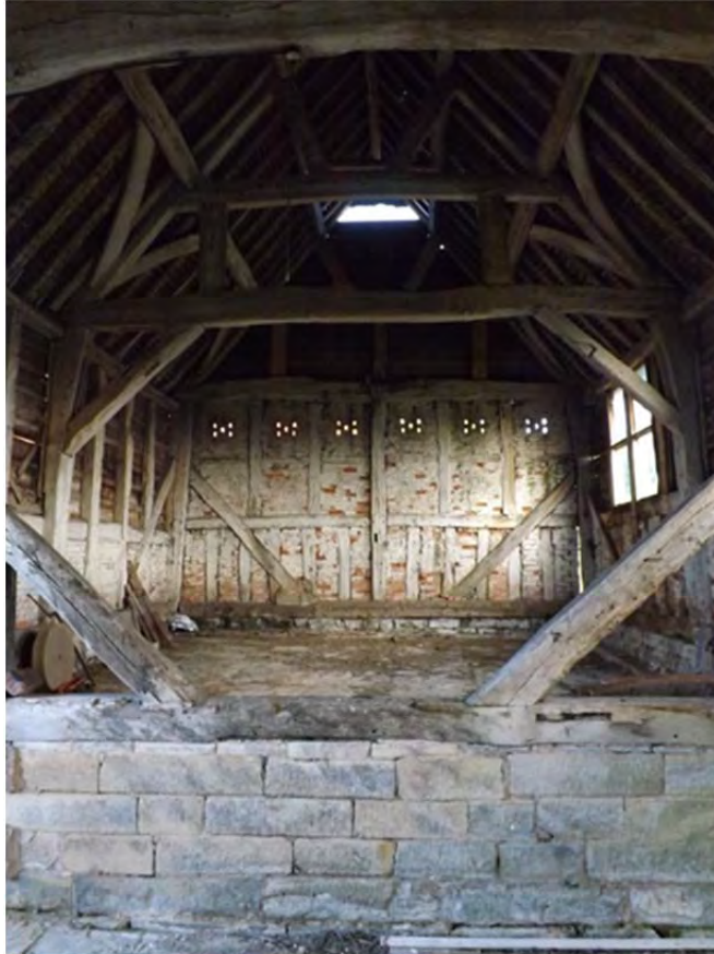
IBC 15: Barn, north end interior
