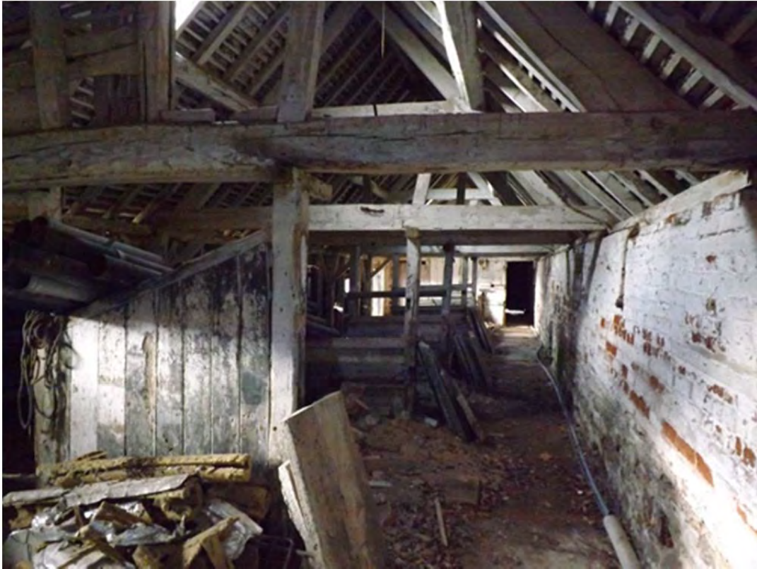
IBC 21: The byre, interior looking west; note the slope of a re-used stable travis to the left
