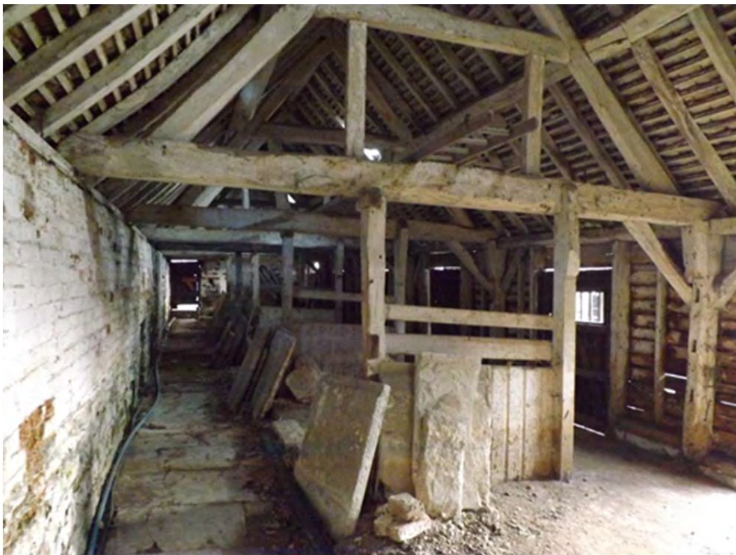
IBC 20: The byre, interior, looking east
