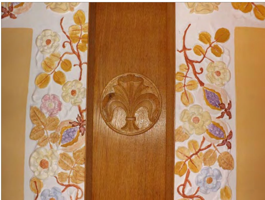
IBC 10: Parquetry (not normally painted) and carved detail on a ceiling beam
