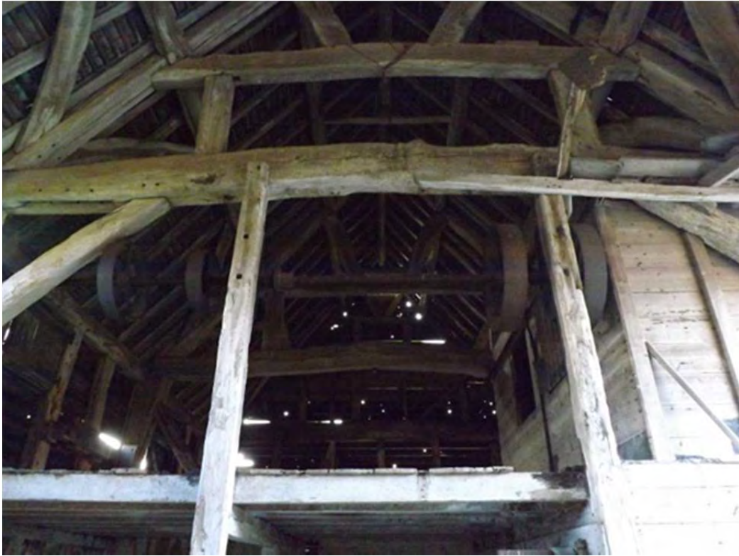
IBC 17: Barn interior, the queen-post roof and belt-driven shaft and wheels
