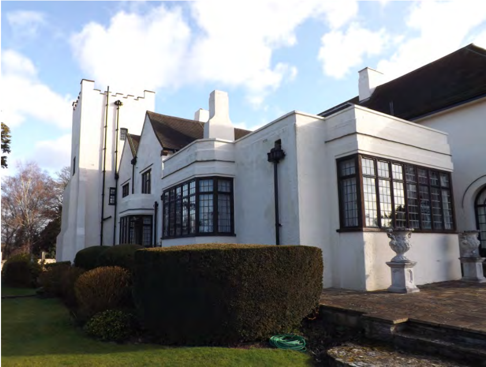
IBC 5: The 1930s Art deco wing containing the Billiard Room; it is currently flat-roofed behind a high parapet (roof level indicated by rain-water hopper)
