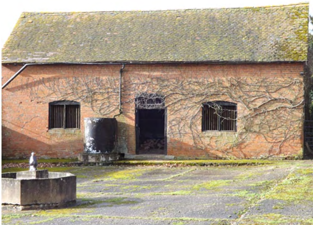
IBC 28: The stable from the farmyard
