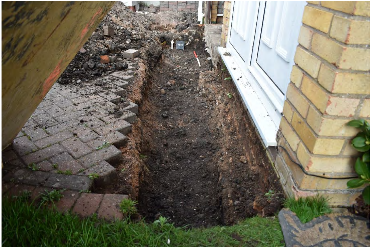
5: Trench to the west of the site, looking north
