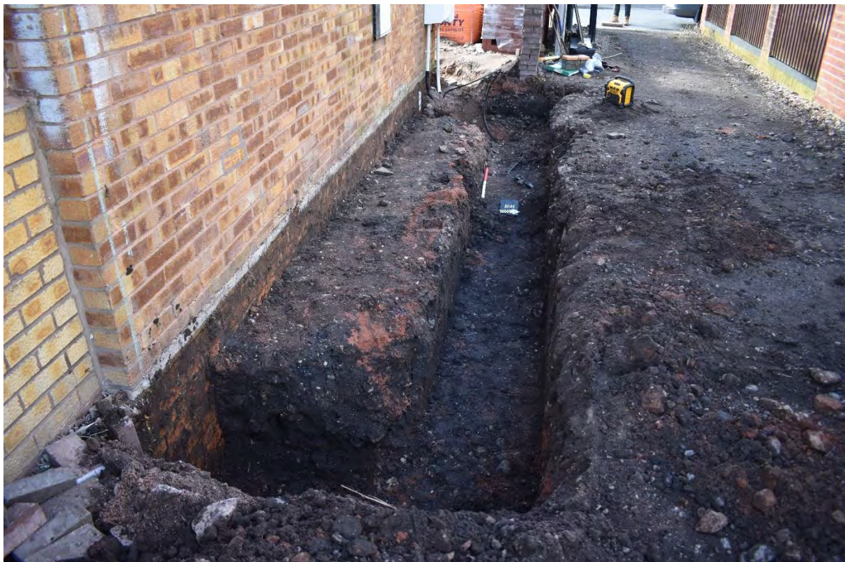
4: Trench at north of the site, looking west
