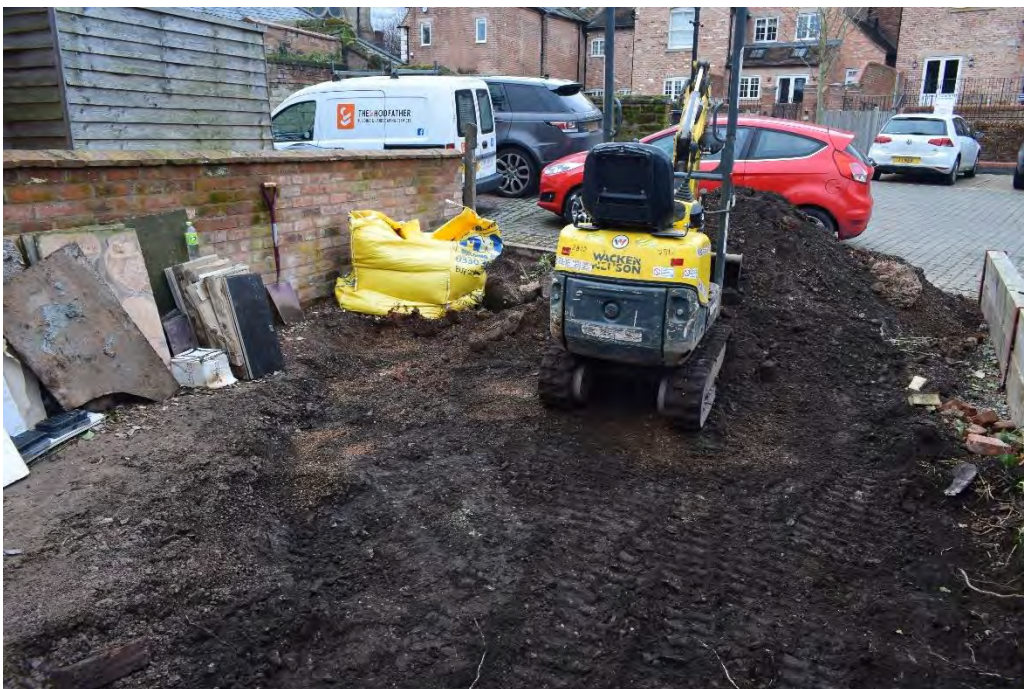
10: General shot of site post-excavation, looking south
