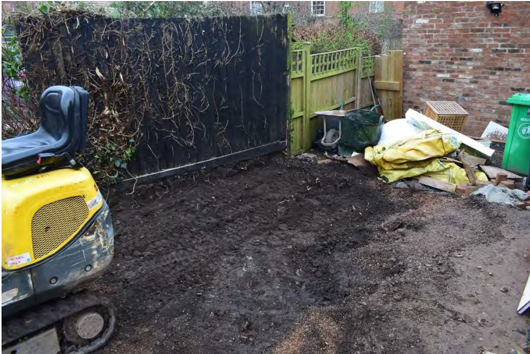
9: General shot of site post-excavation, looking north
