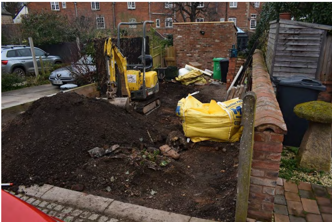
8: General shot of site post-excavation, looking north
