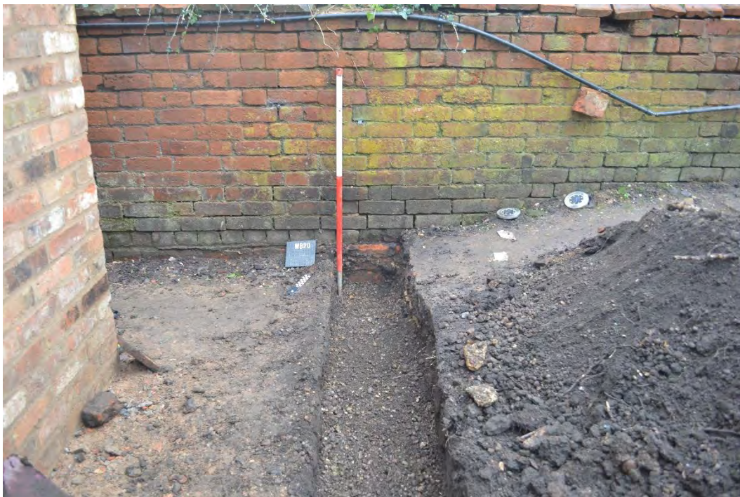
2: Trench for retaining wall, looking SE
