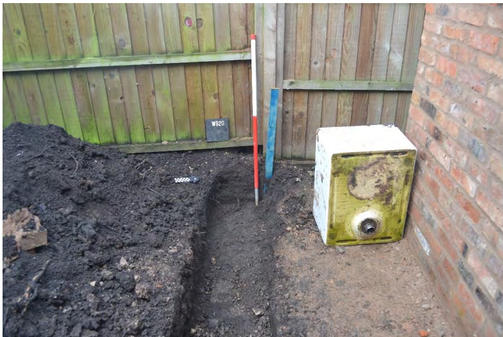
4: Trench for retaining wall, looking NW
