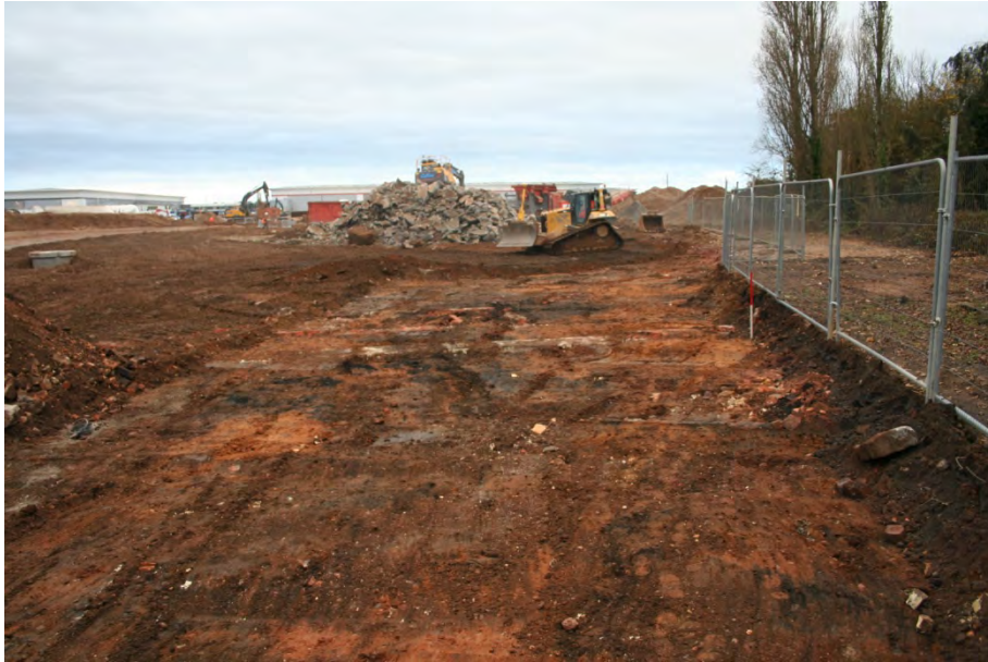
7. Ground reduction looking south-east
