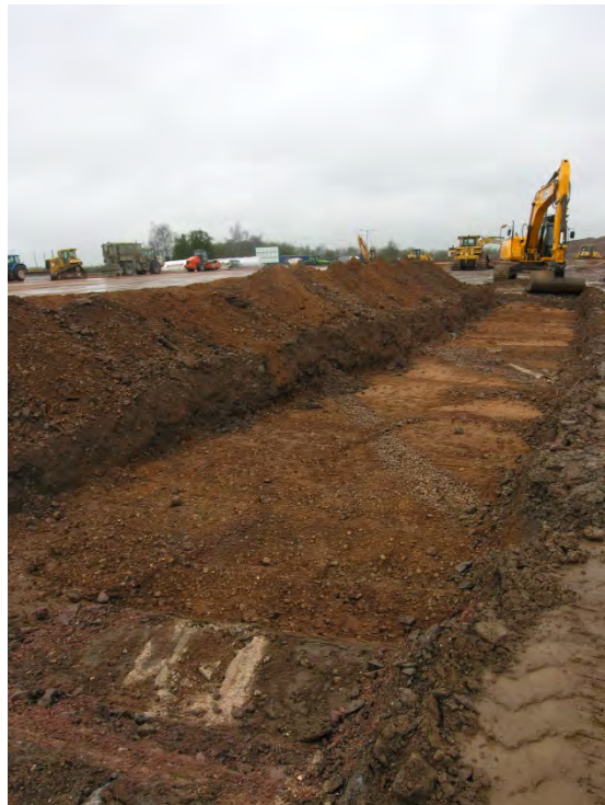
2. Ground reduction showing intrusive concrete and drainage cuts in 2014
