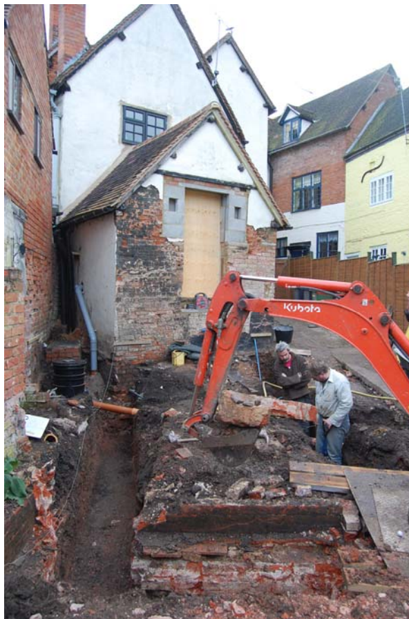
Fig 3: Trenches being excavated and the rear of Red Horse House
