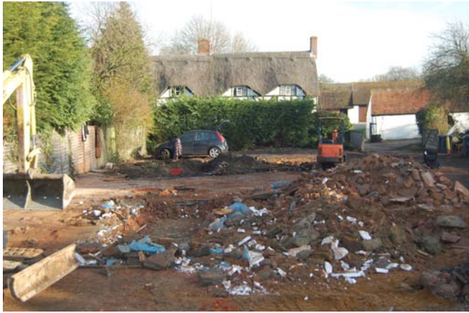
Fig 6: View eastwards across site
