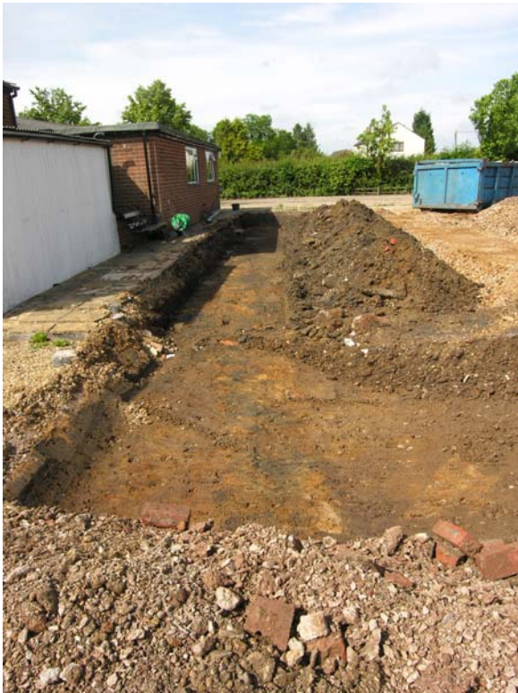
Fig 7: The south arm (rectangular trench)
