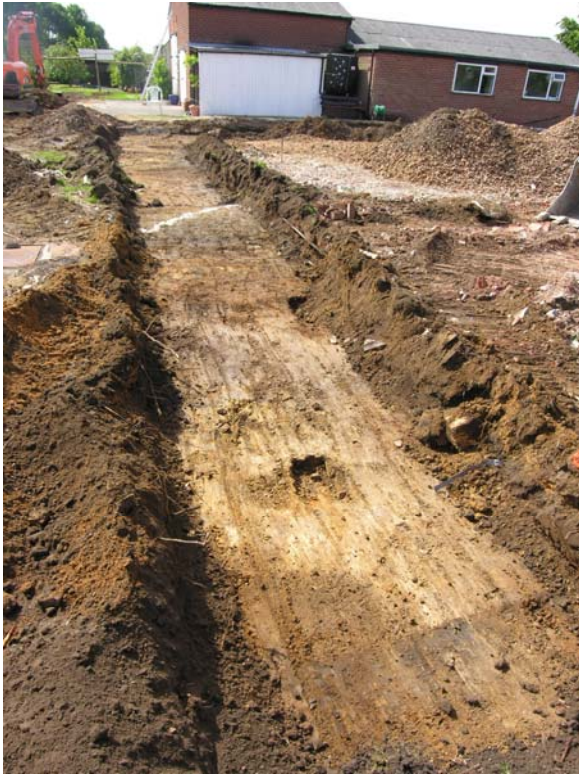
Fig 5: The east arm (rectangular trench)
