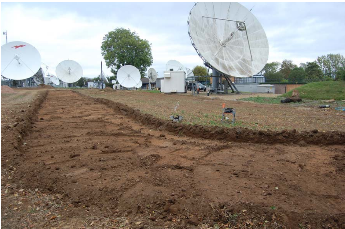
Fig 7: New access road viewed from the SW
