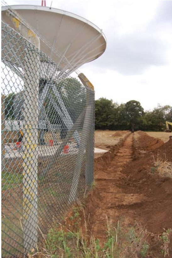
Fig 5: New fence trench from the NE
