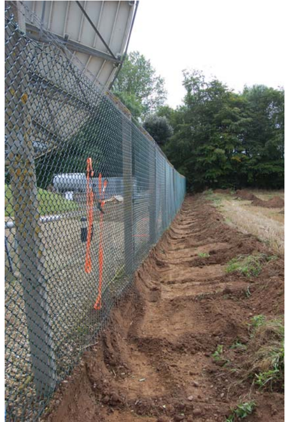
Fig 6: Old fence trench from the NE
