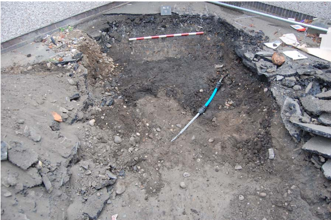
Fig 6: Trench 1 showing location of broken lead water pipe viewed from the north
