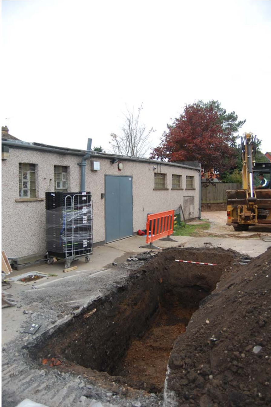
Fig 7: Trench 2 viewed from the NNE
