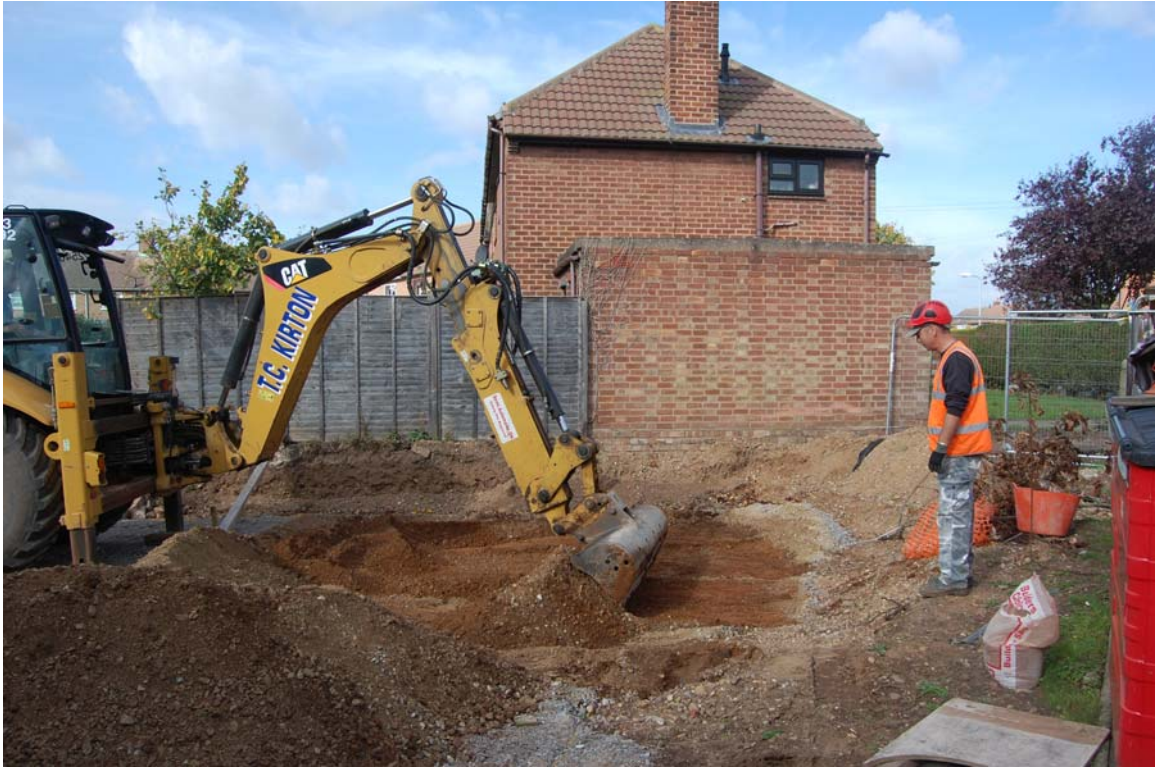
Fig 5: Removal of temporary hard-standing in progress
