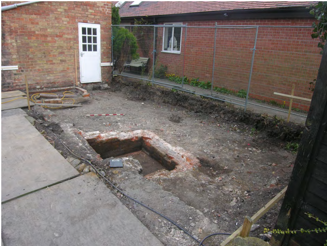
Fig 7: Area observed, looking north
