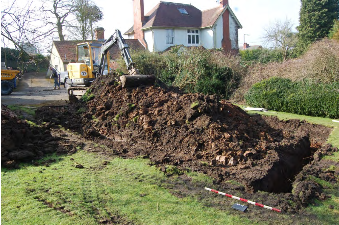
Figure 5: Excavation of garage trenches
