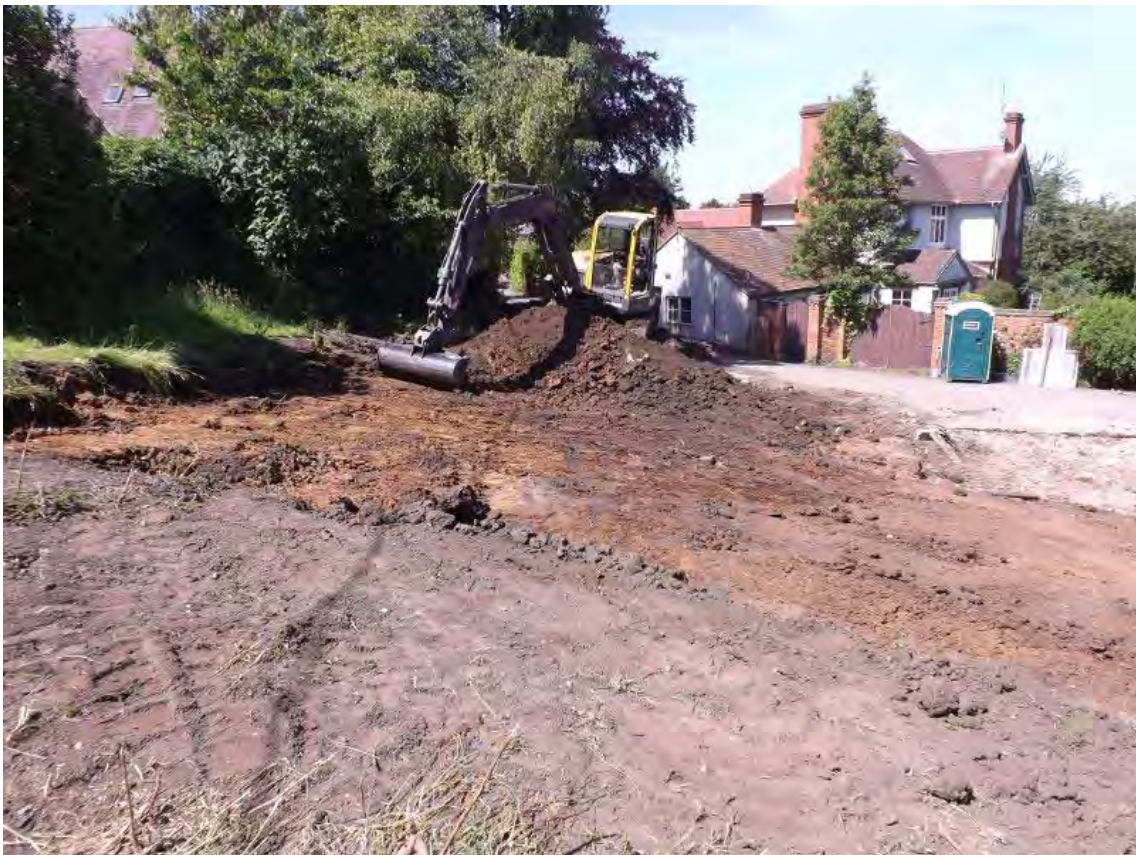
Figure 6: Ground reduction for new house
