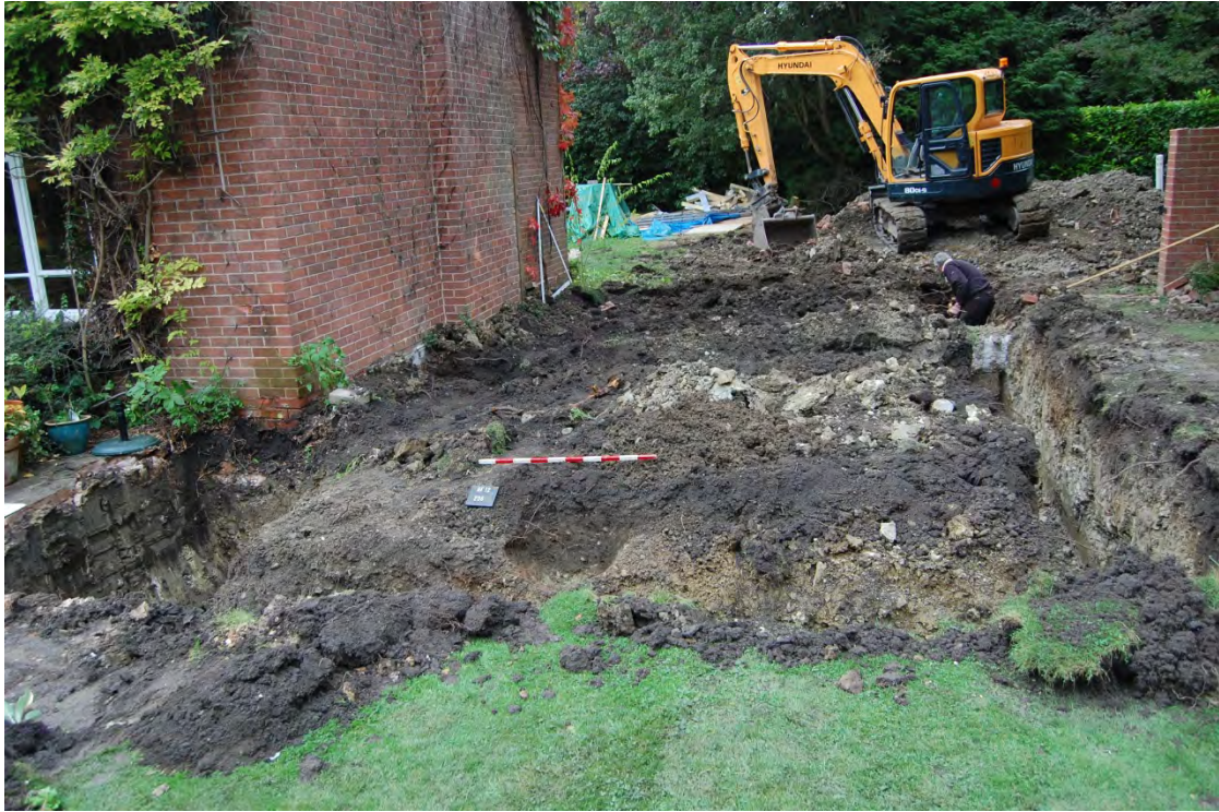
Fig 7: Area 2, new extension, looking north
