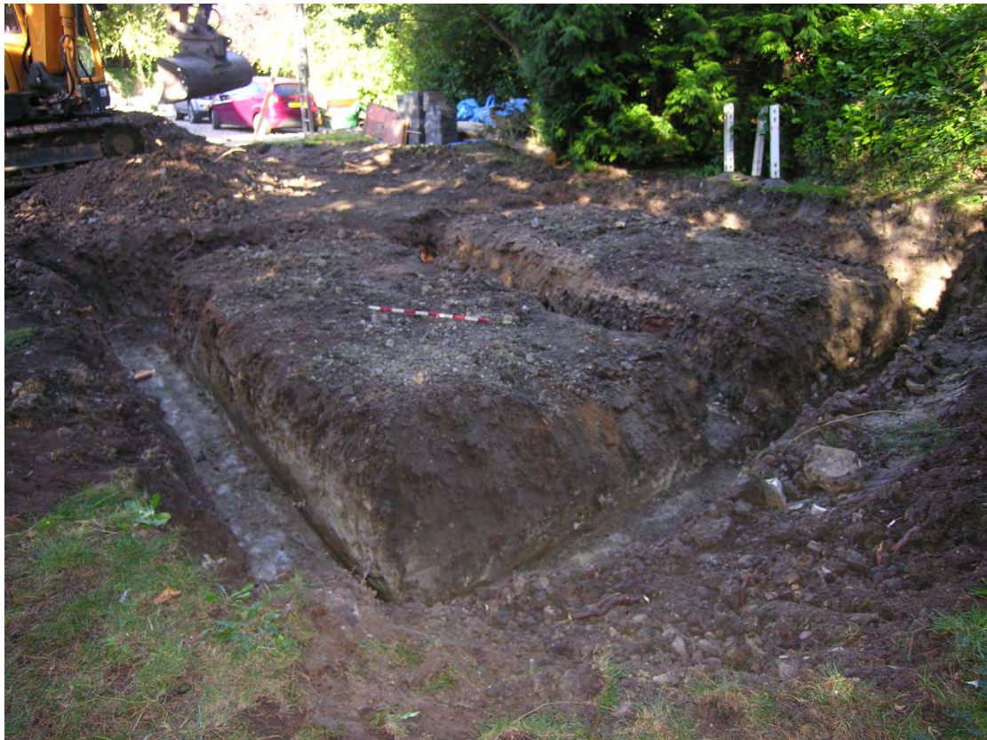
Fig 8: Area 3, new garage, looking north-west
