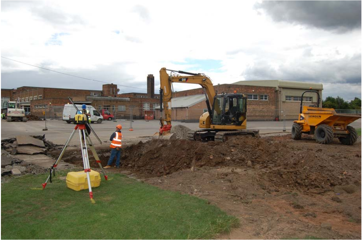
Fig 7: Soil stripping for proposed sports pitch
