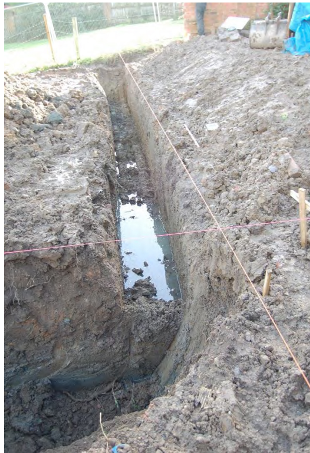
Fig 6: Foundation trench at west end of the site
