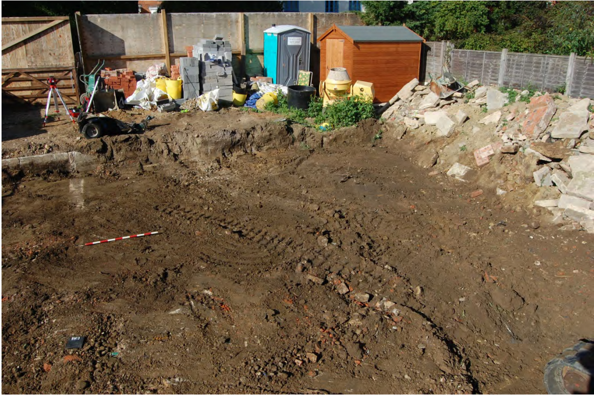
Fig 5: Initial soil stripping of western part of the site
