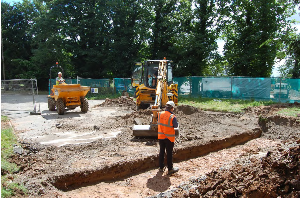
Fig 5. Trenching in progress
