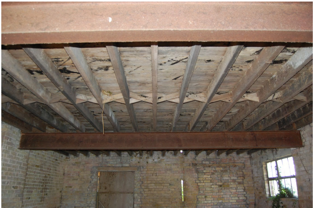
Fig 10: Interior of barn, granary floor
