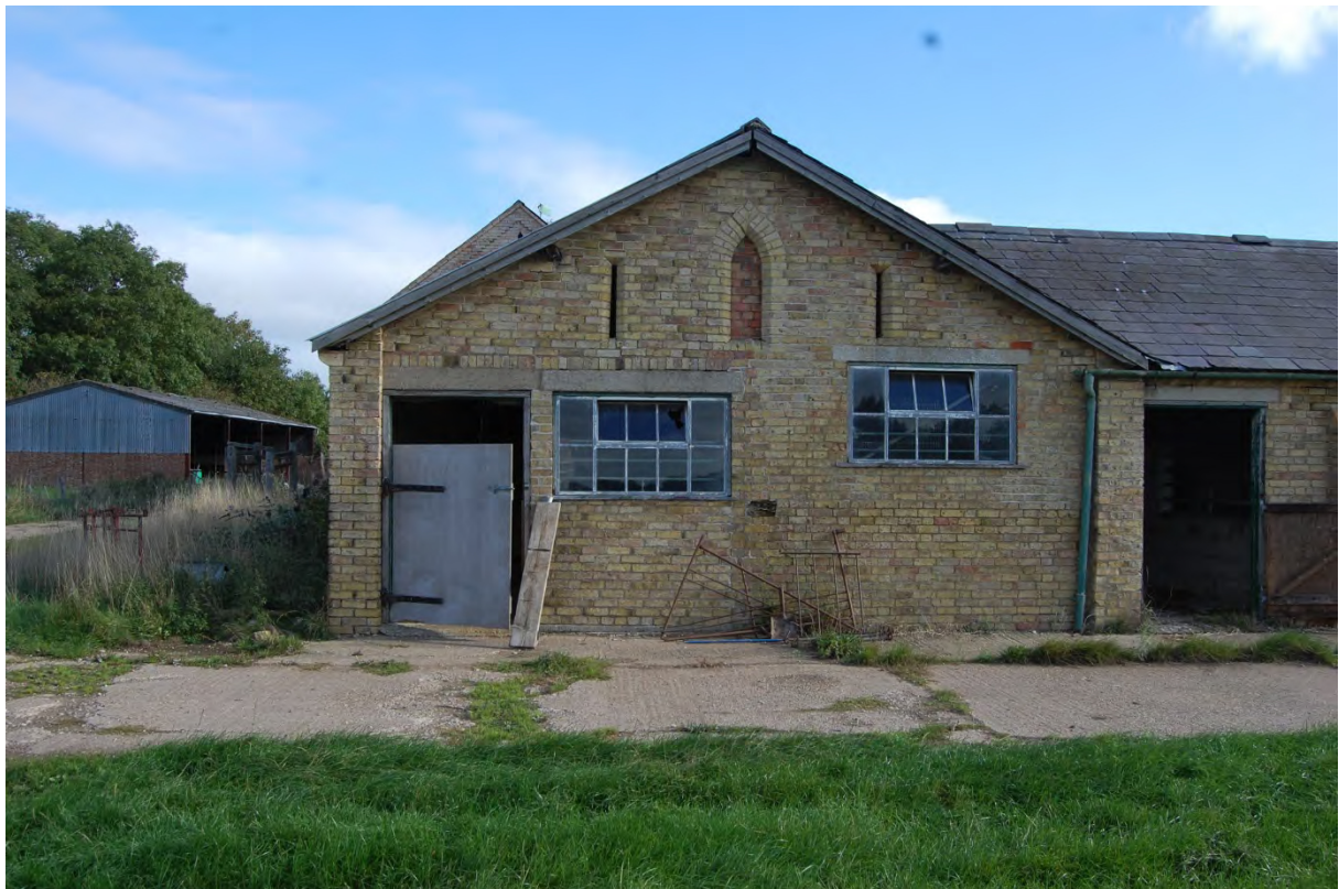
Fig 21: Gable end of western building
