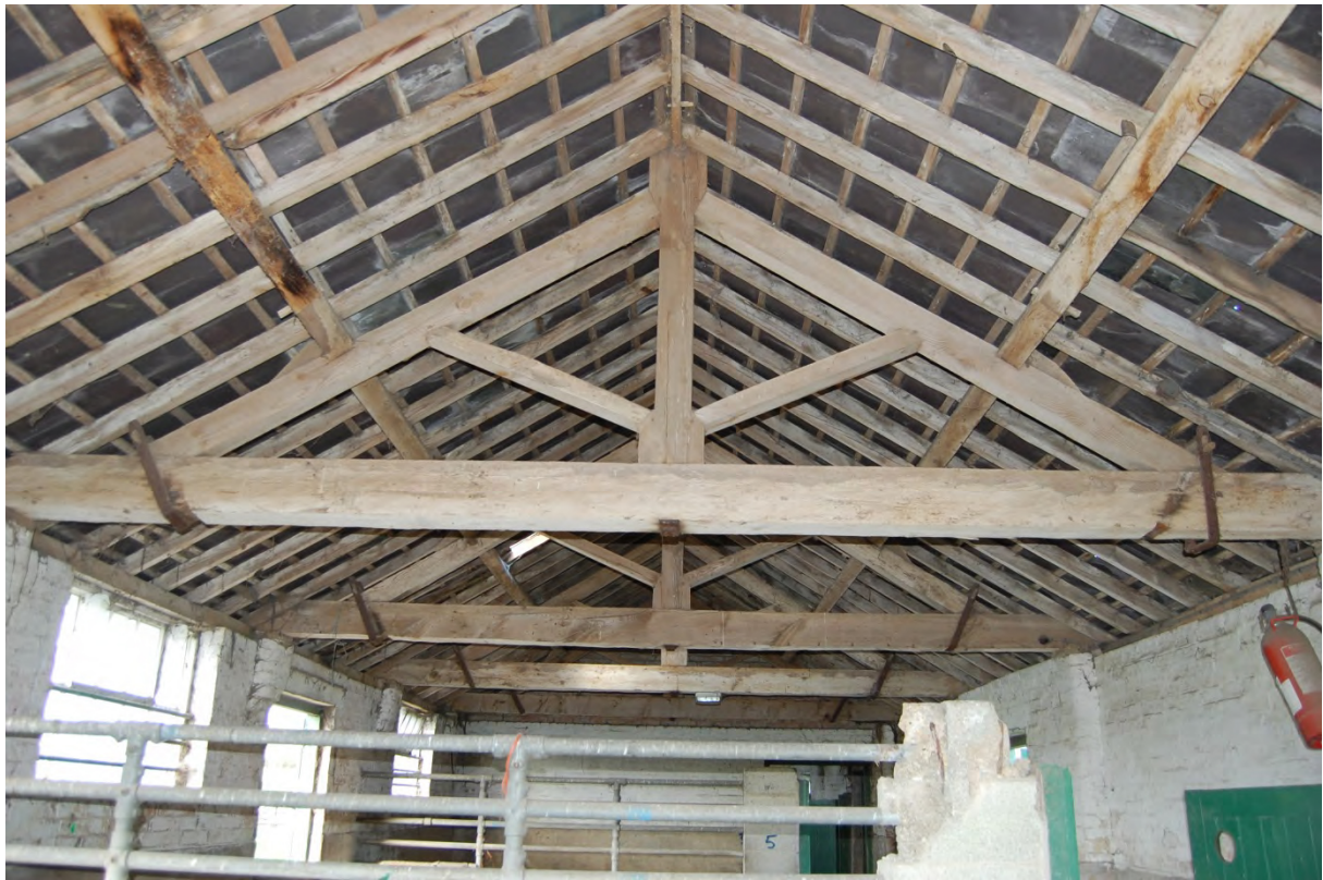
Fig 20: Roof structure of SW range (T/U)
