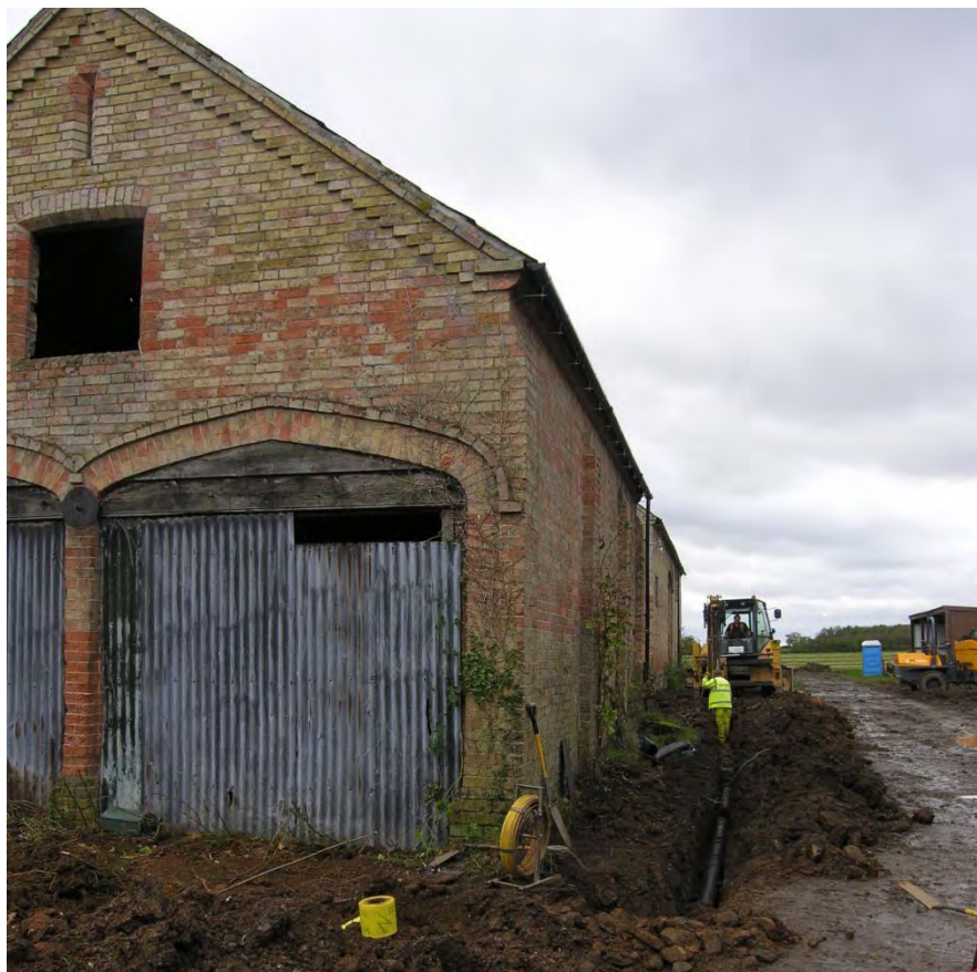
Fig 25: Service trench to rear of coach house
