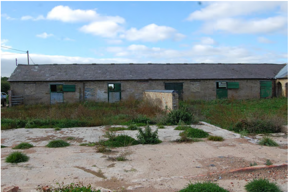
Fig 18: Former milking parlour (SW range)
