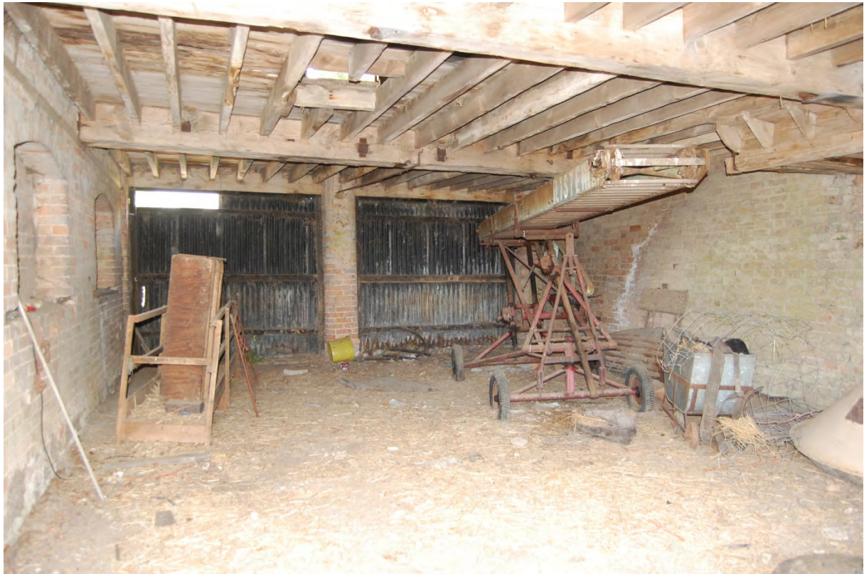
Fig 16: Interior of coach house (I)
