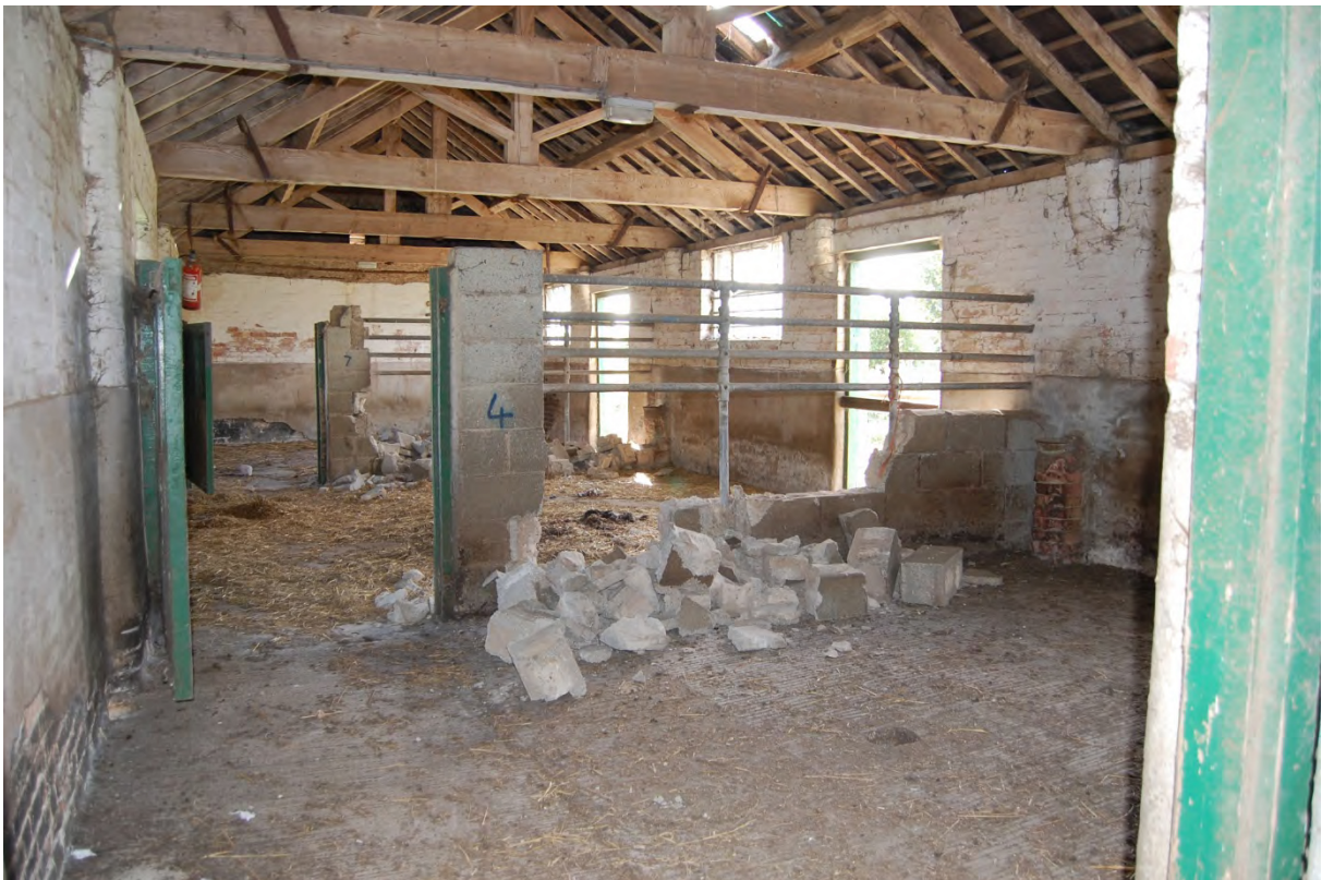
Fig 19: Interior of SW range with part demolished internal walls (U)
