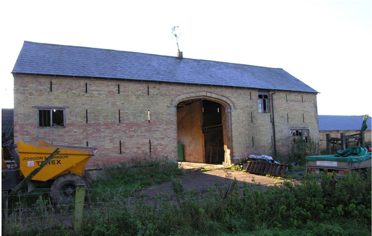
Fig 9: Rear of threshing barn
