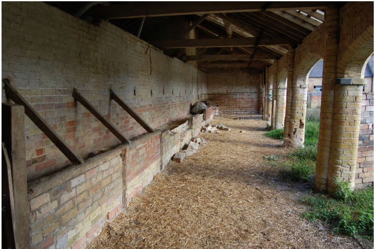
Fig 22: Open-fronted shelter shed (Q)
