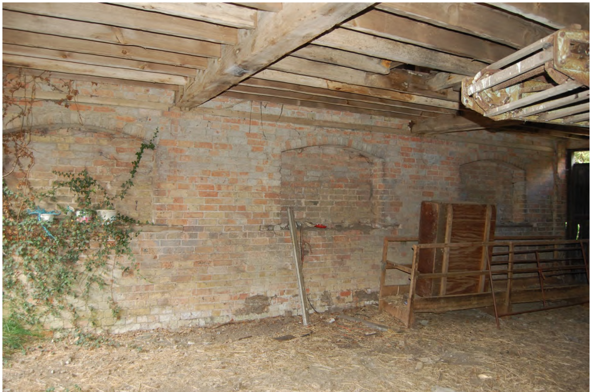
Fig 17: Interior of coach house (I)
