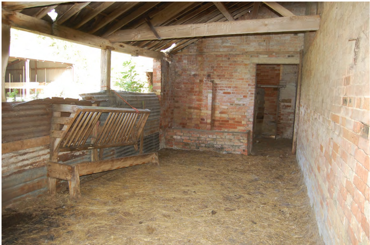
Fig 23: Shelter shed (L)
