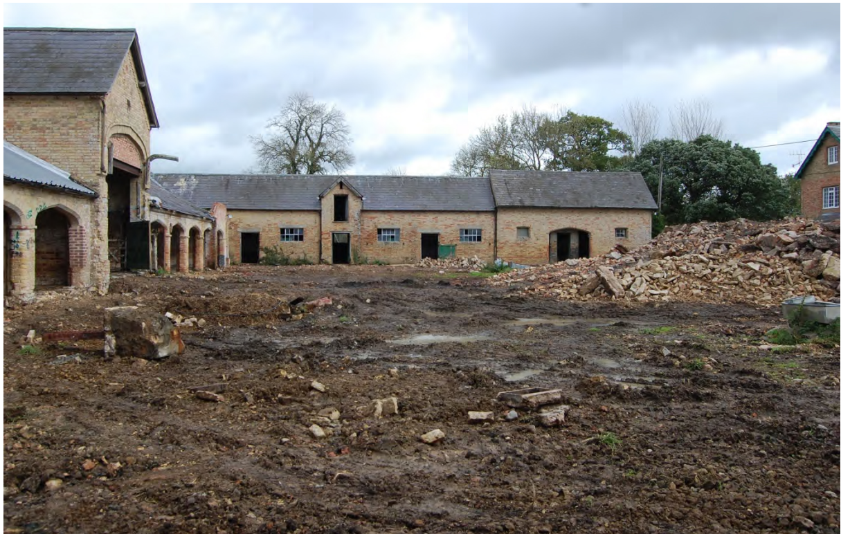
Fig 24: Courtyard after demolition of walls and breaking up of concrete
