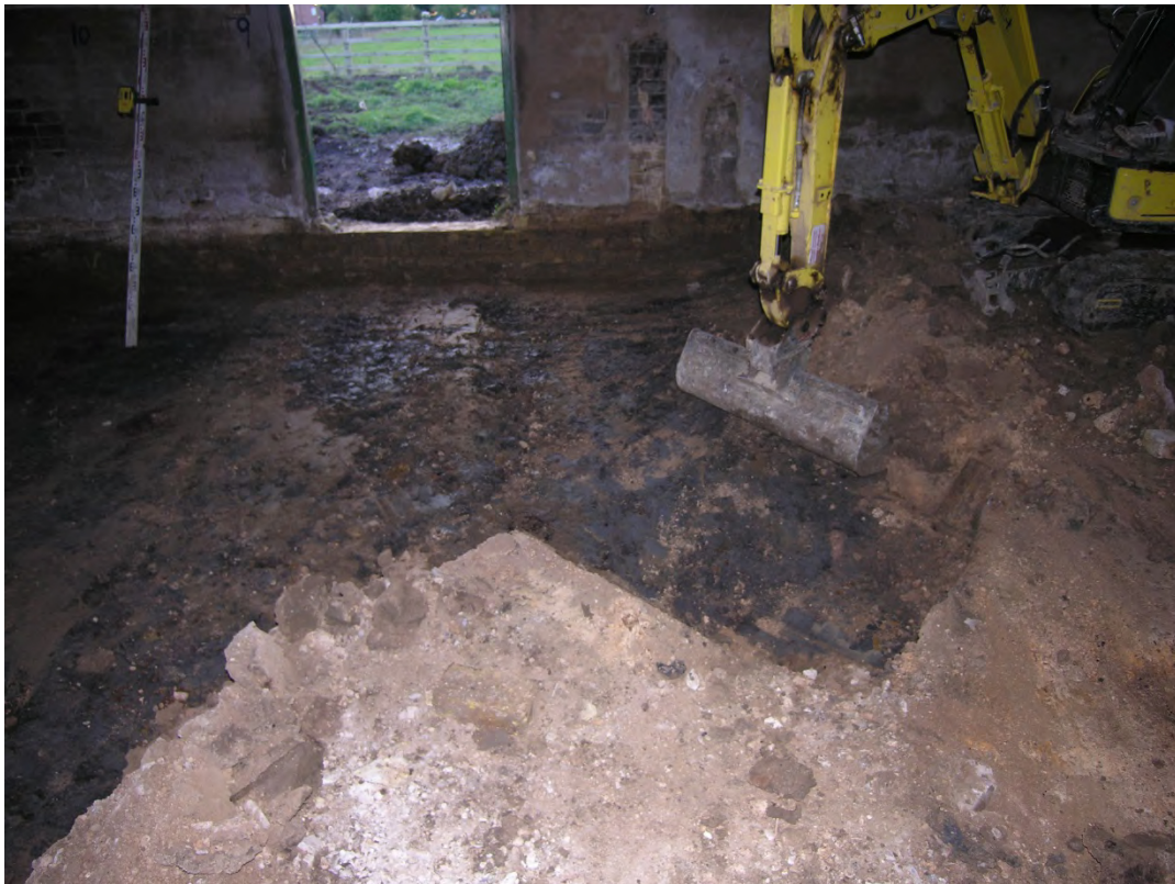
Fig 26: Ground reduction within SW range
