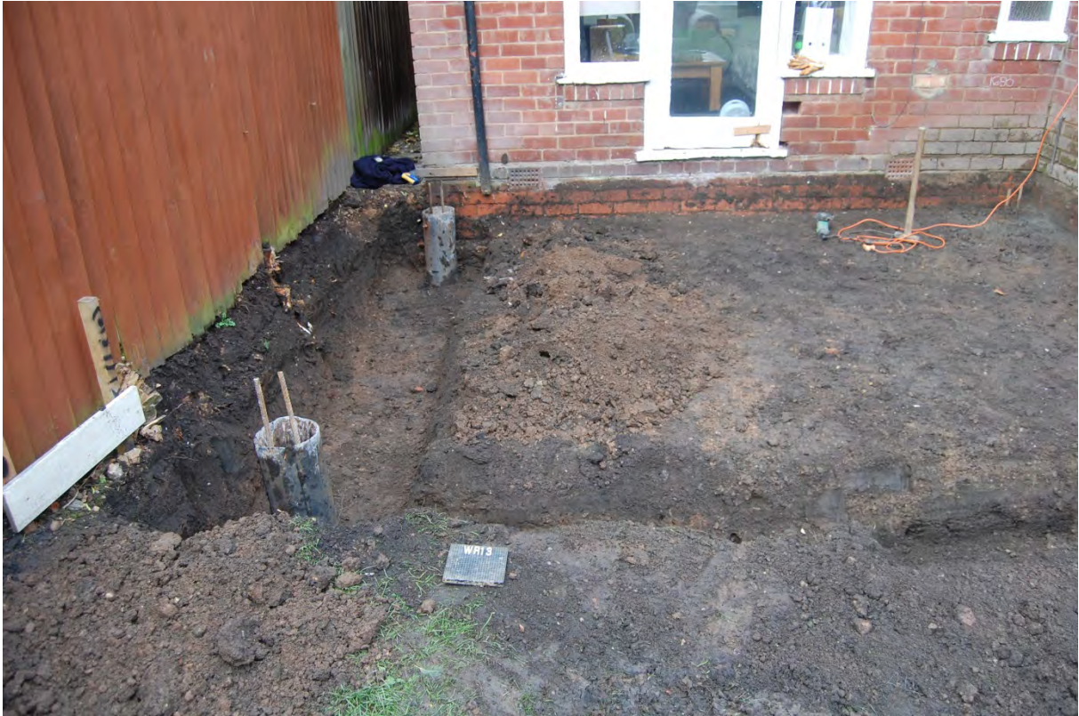
Fig 7: The site reduced and trenches excavated
