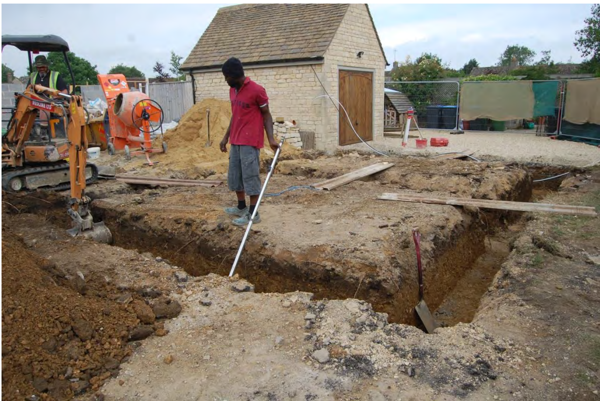
10. Excavation of trenches for new garage
