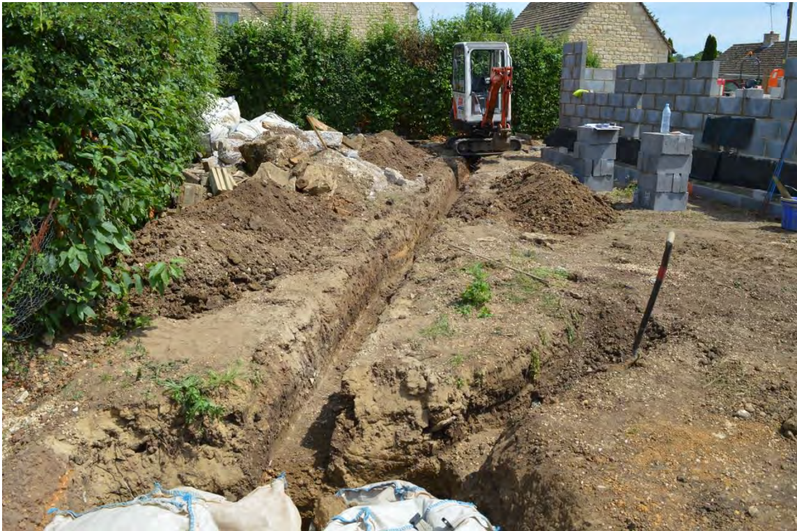
9. Excavation of ST3 and ST4
