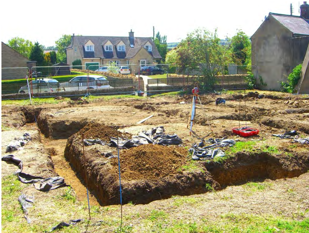
1. General view of foundation trenches excavated for new house
