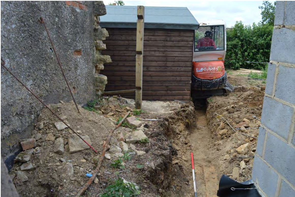
7. Brick wall 132 in ST2 with rubble 130 of stone walling
