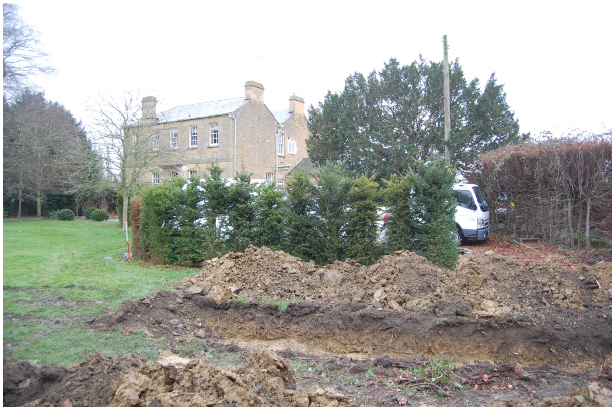
Fig 6. The trench in relation to The Old Rectory
