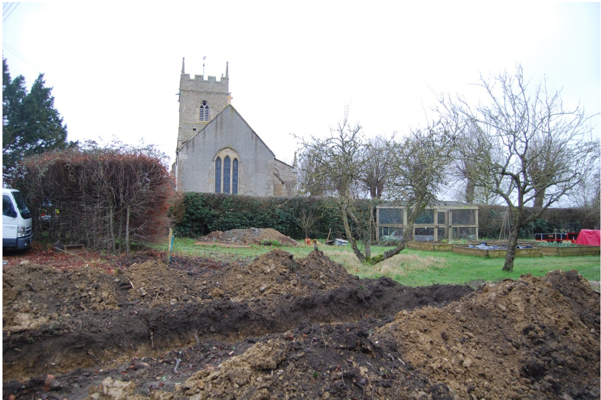
Fig 5. The trench in relation to the church
