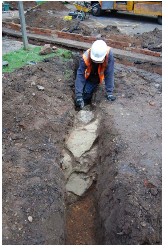
Photograph 3: Wall 30 being cleaned
