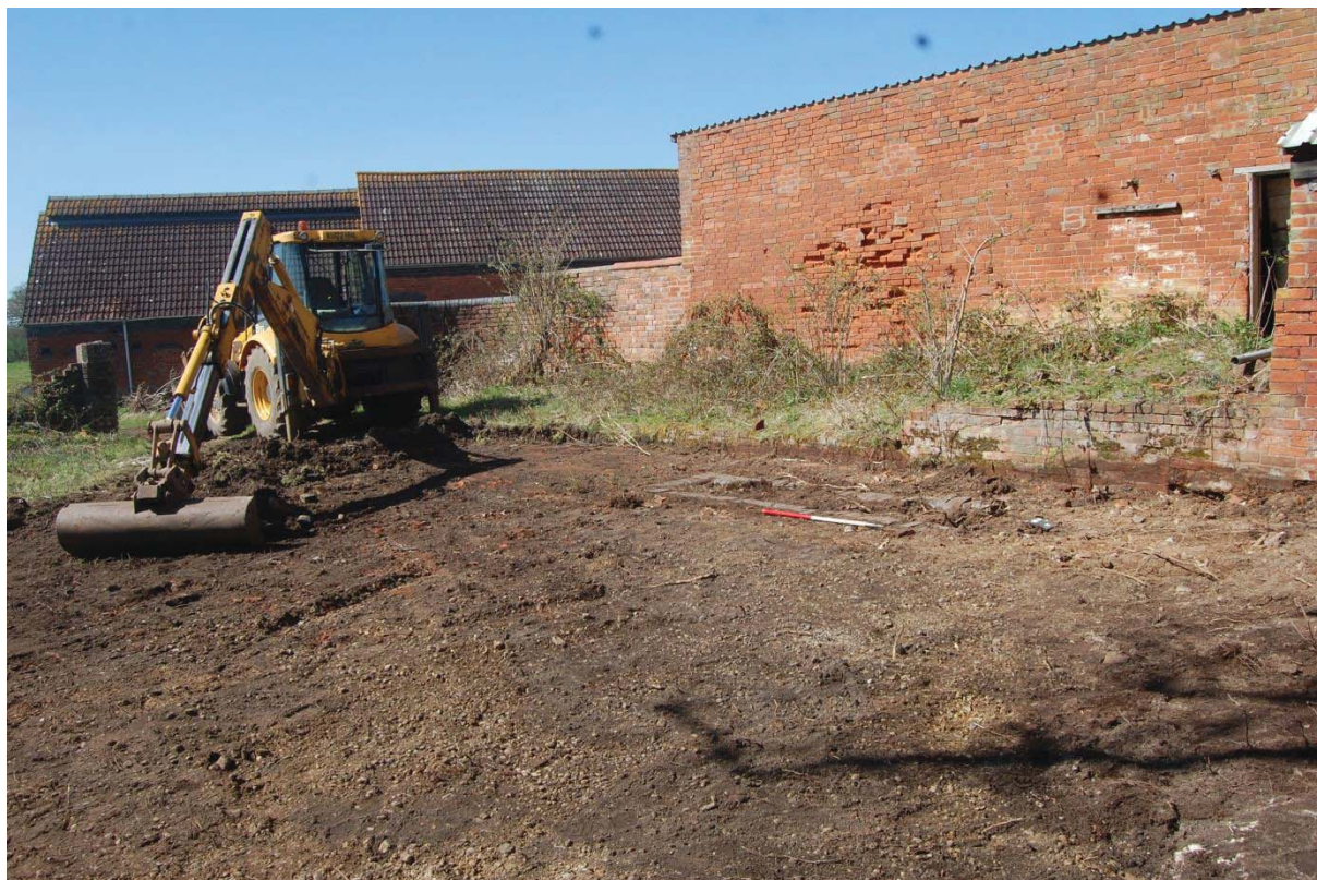
6: Ground reduction taking place, brick-lined pit (29) exposed
