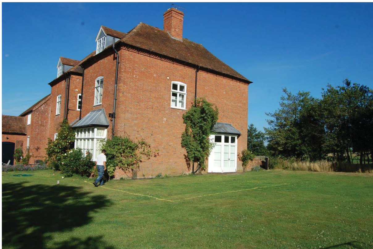
2: North-west side of present house before groundworks
