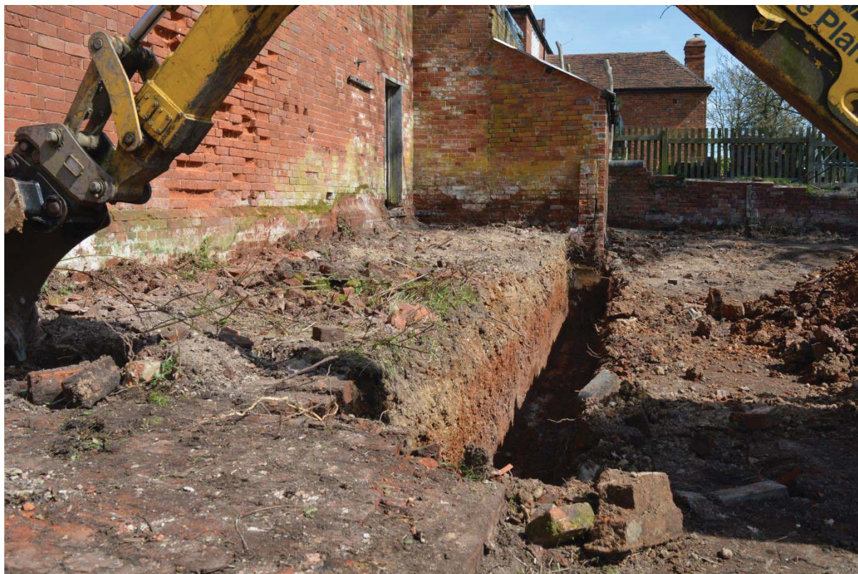
8: Trenching for new extension
