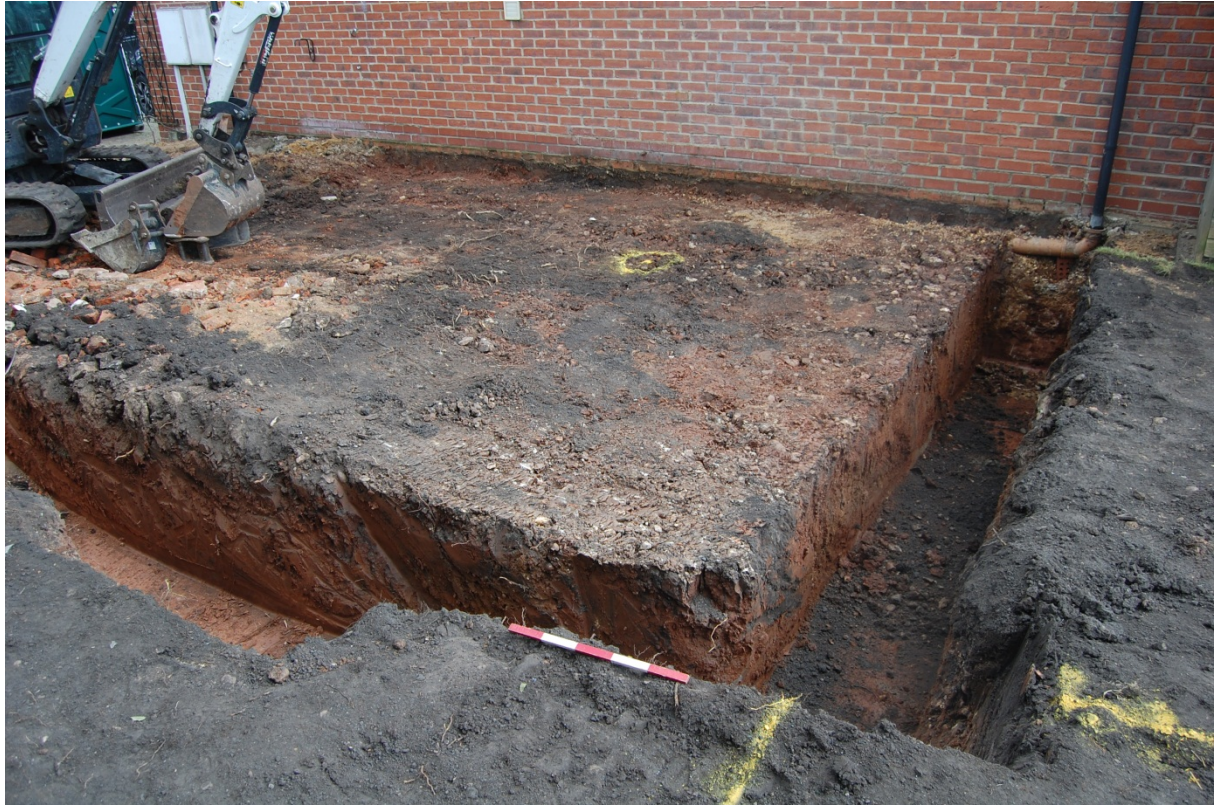
Fig 4: Trench, looking SE
