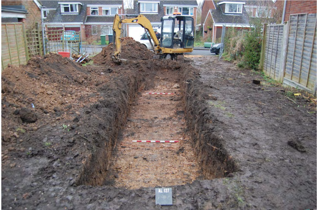
Fig 4: Evaluation trench viewed from the north
