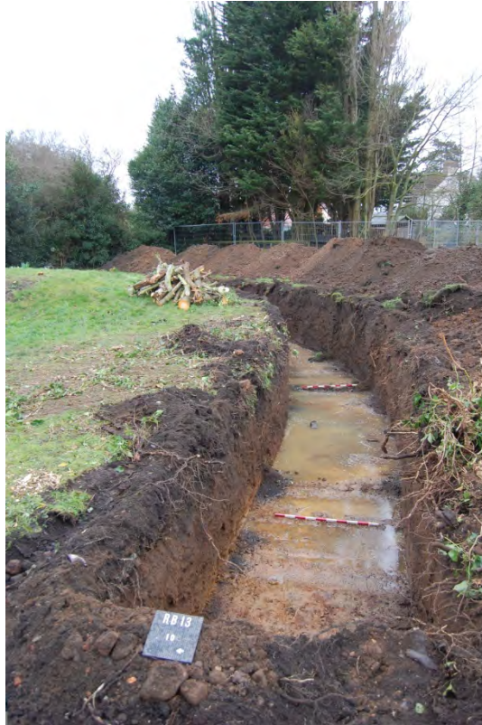
Fig 10: Trench 10, looking East
