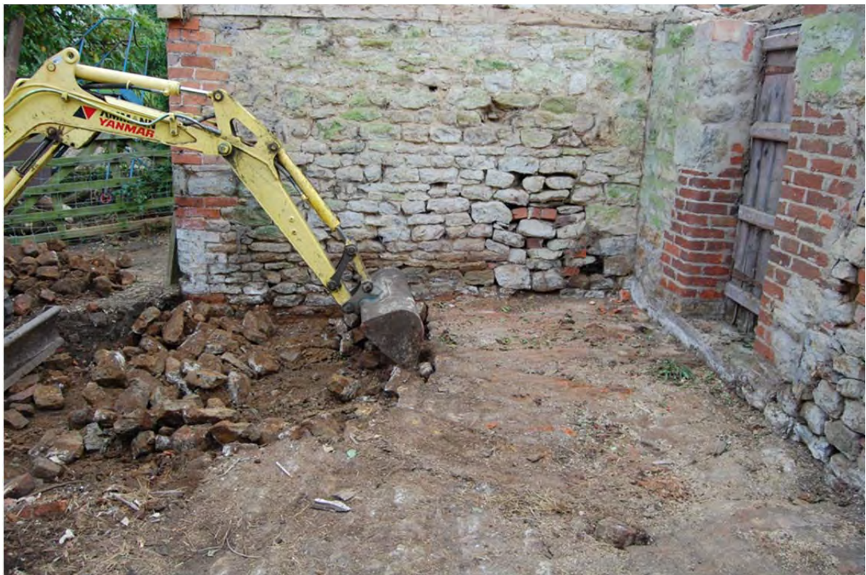
Fig 6: Removal of composite floor of barn
