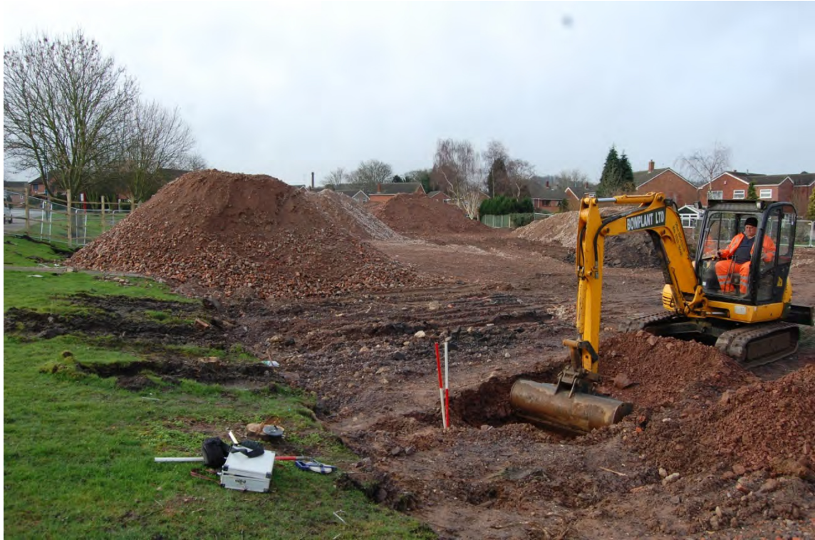
Fig 5: General view of site looking south-west
