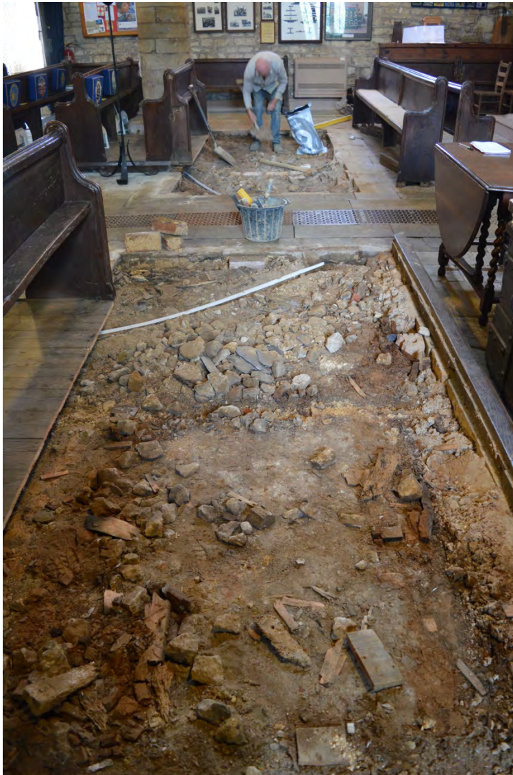
Fig 2: Rubble (6) exposed below floor boards
